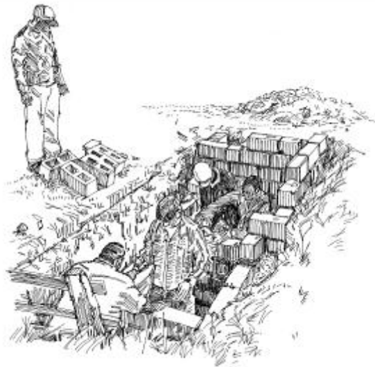
Lining a latrine pit (Credit: Shaw, 2005)
