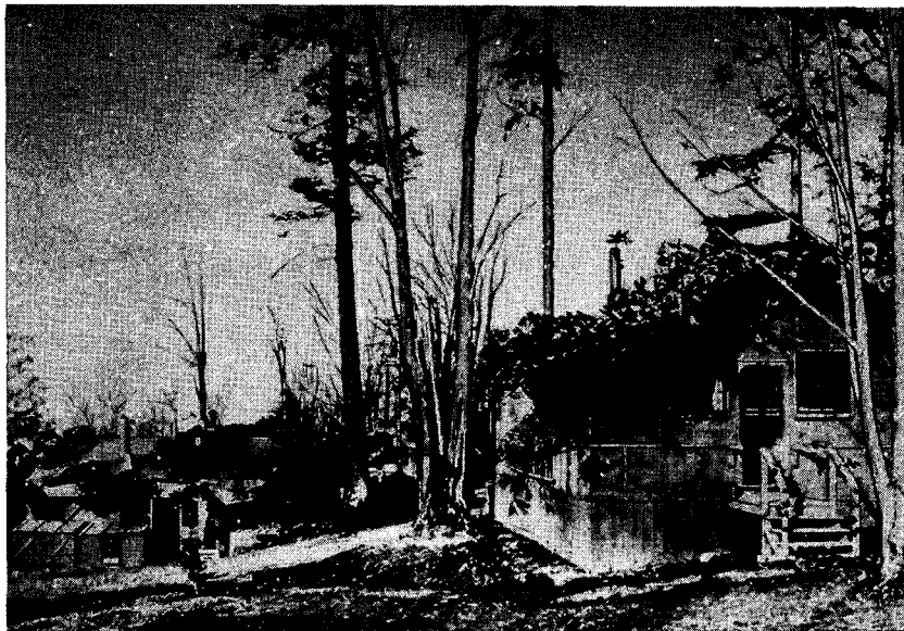
Figure 58. Another method of breaking identifying shadows is to attach silhouettes of plywood or other rigid materials to the eaves.
