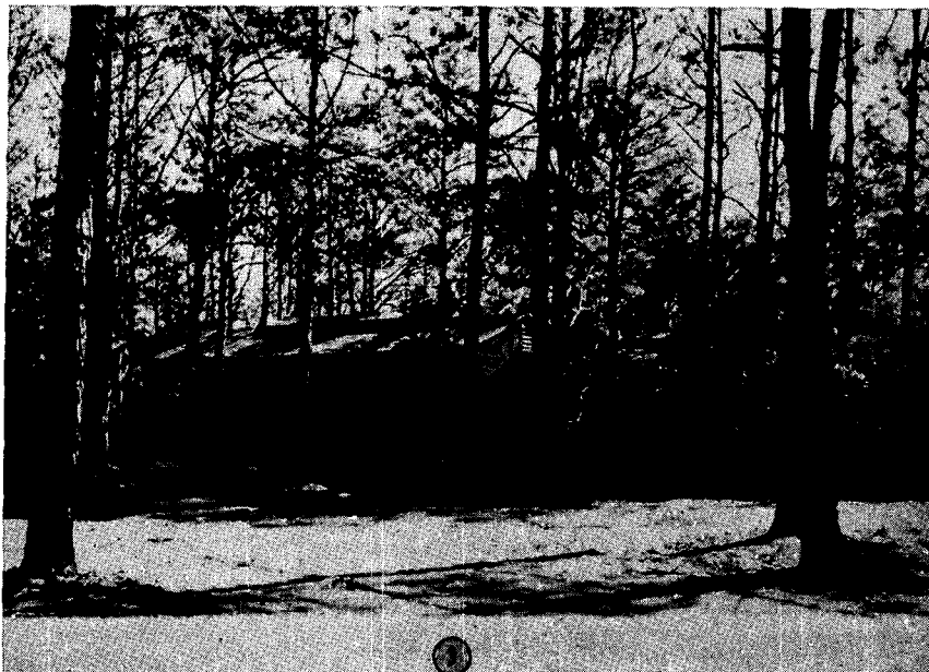
Figure 70. Closeup view of barracks shown in ②, figure 69.
