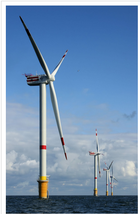
The natural resource of wind powers these 5MW wind turbines on this wind farm 28 km off the coast of Belgium.
