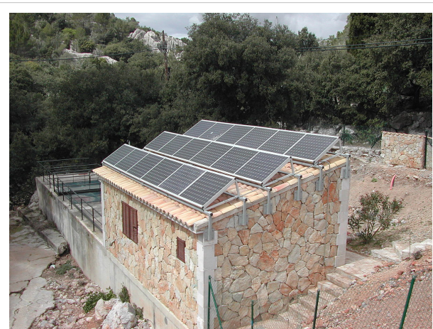
A sewage treatment plant that uses environmentally friendly solar energy, located at Santuari de Lluç monastery.
