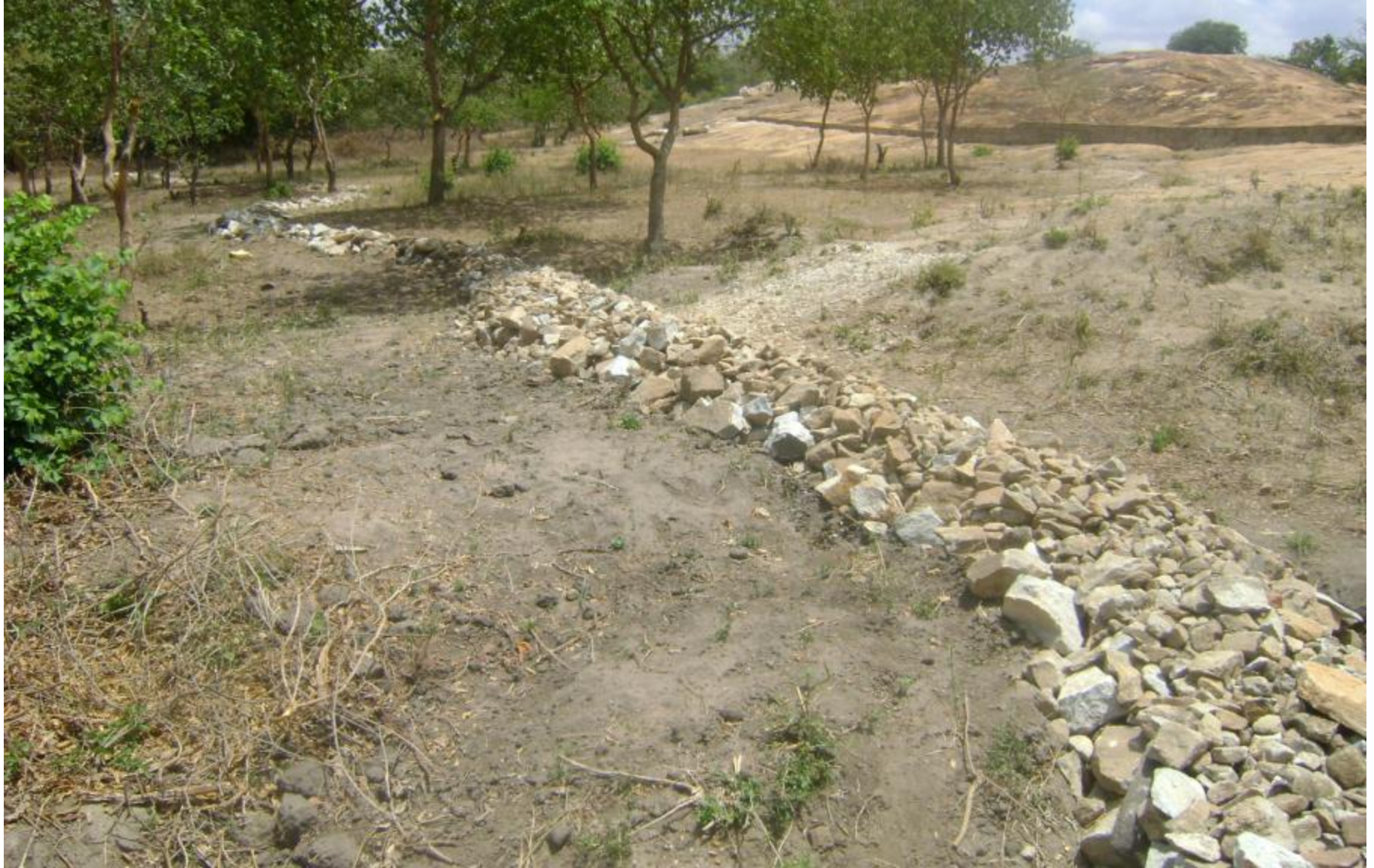
Permeable rock check dams for gully control and catchment conservation in a water project site, Makueni district
