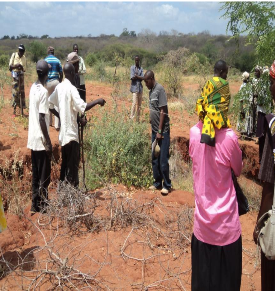
Measuring slopes and marking contours using line level
