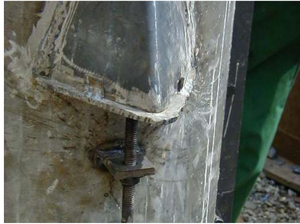
Insert the nose plate and lock it into place using the bolt.
