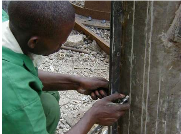
Unscrew the bolts from the sides of the outer shells.
