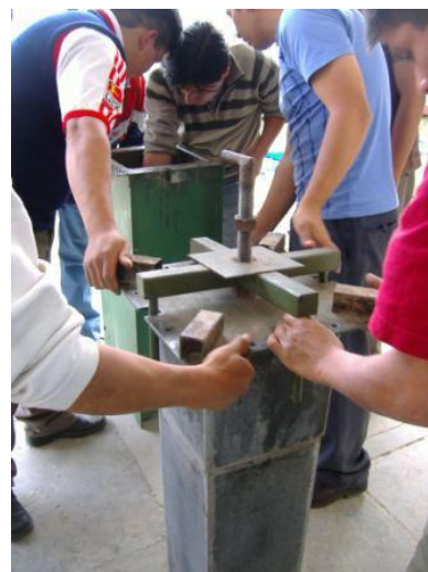
Figure 4: Removal of the concrete filter from the metal mould. Photo: Soluciones Prácticas.
