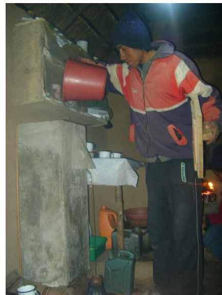
Figure 2: A domestic bio-sand water filter being used in Peru. Photo: Soluciones Prácticas.
