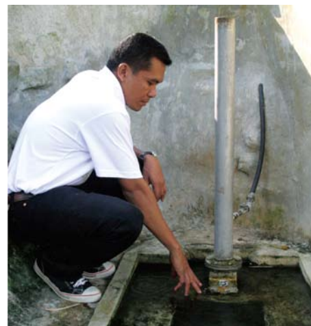
Checking the ram pump intake
