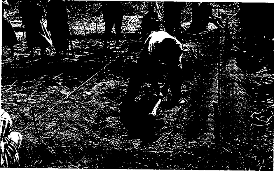
Leveling a basin by eye using a khasu
