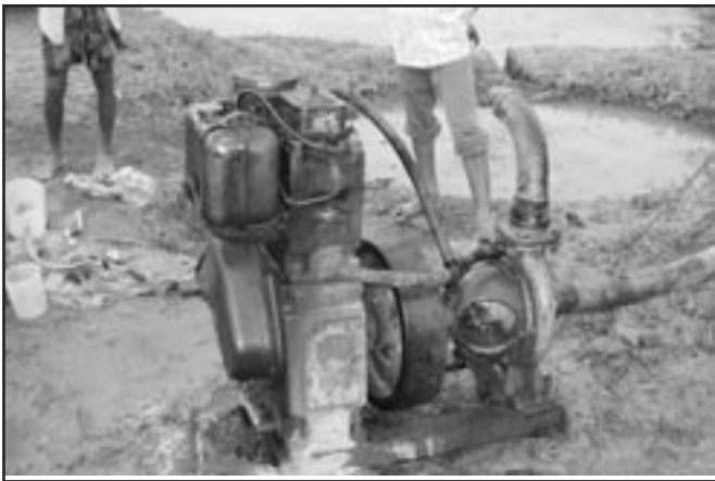
Photo-3: Ten years old diesel pump in Panishala, Cooch Behar I block
