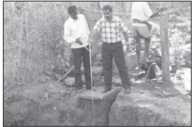
Photo-8: Measuring of Depth of well in Tellanpalli village, Balangir district, Orissa
