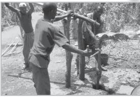
the hole. This technique allows the drill bit to scrape compact layers of sand, clay, sand stone or tuff stone. It does not work with solid rocks.
