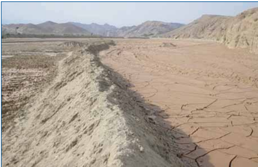
FIGURE 4.4 Traditional spate irrigation intake in Pakistan
