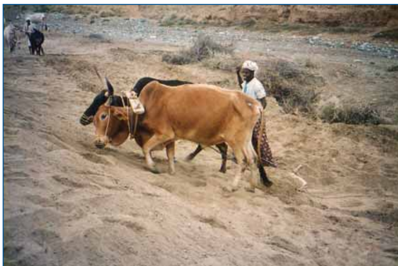
FIGURE 5.1 Field bund being strengthened with soil scraped up from irrigated land
