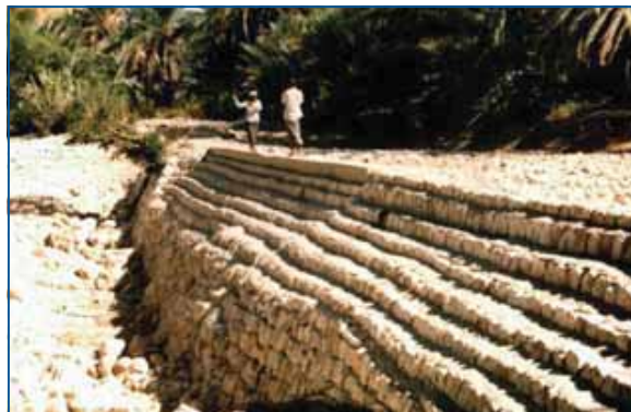
FIGURE 4.8 Diversion weir with stepped downstream face
