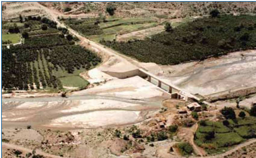
FIGURE 4.15 Wadi Rima spate irrigation intake, Yemen
