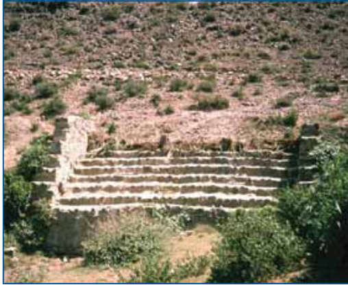
FIGURE 4.12 Side spillway constructed by farmers in Wadi Rima in Yemen
