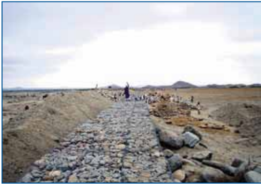
FIGURE 4.10 Rehabilitated traditional weir in Wadi Hadramawt
