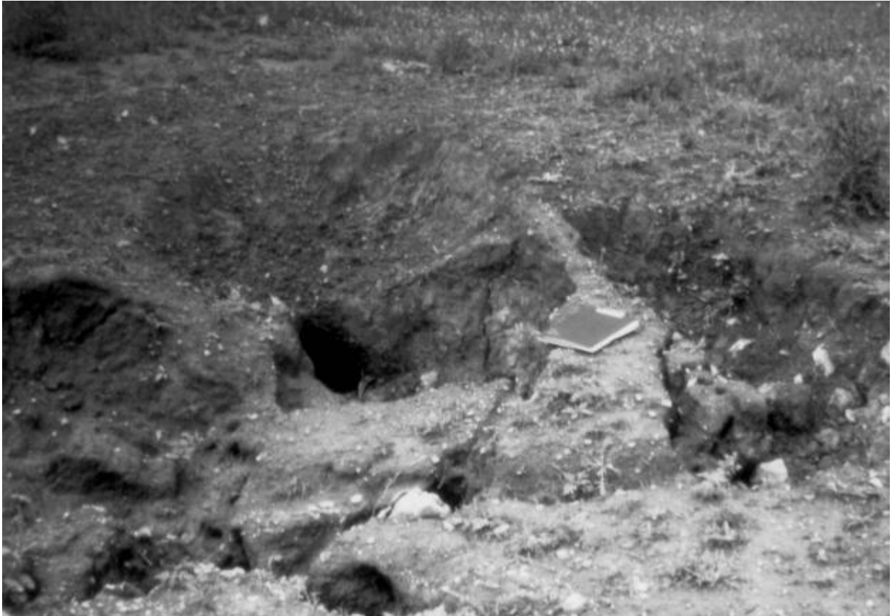
Photo of a sinkhole formed in karst soil.
