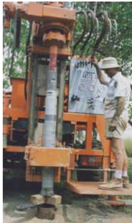
Down the hole hammer with button bit attached
