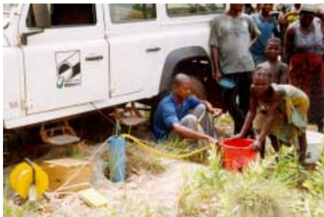
Figure 6.4 Carrying out a pumping test using Whale pumps powered from a car battery.
