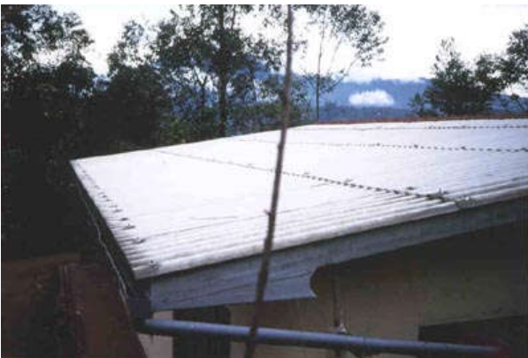
Figure 1: A typical corrugated iron sheet roof, showing guttering. Photo: Practical Action
