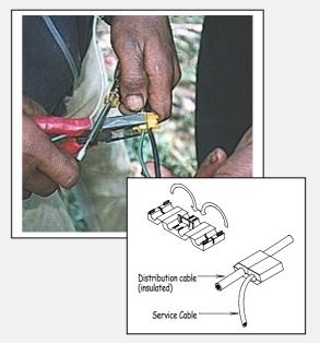
Figure 14-9 and Figure 14-10: Use of a tap splice to connect the service cable to an insulated distribution cable
