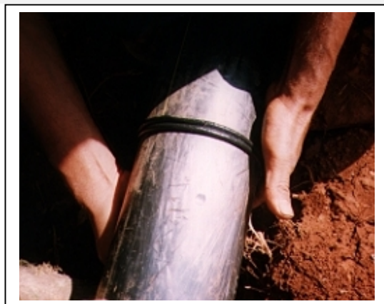
Figure 11-9 The plate is removed and the two sections are brought together forming a neat bead around the pipe.
