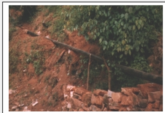
Figure 11-5 Pipe sections that span gaps must be supported at the correct height.
