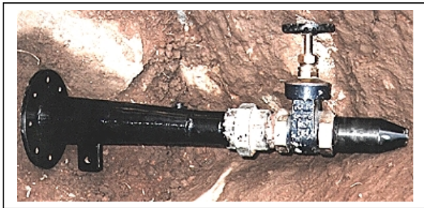
Figure 11-2 Reducer, gate valve and nozzle
