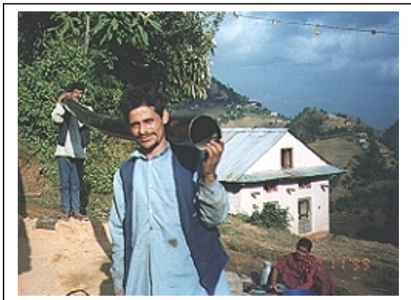
Figure 11-3 Delivering pipe sections to the site.
