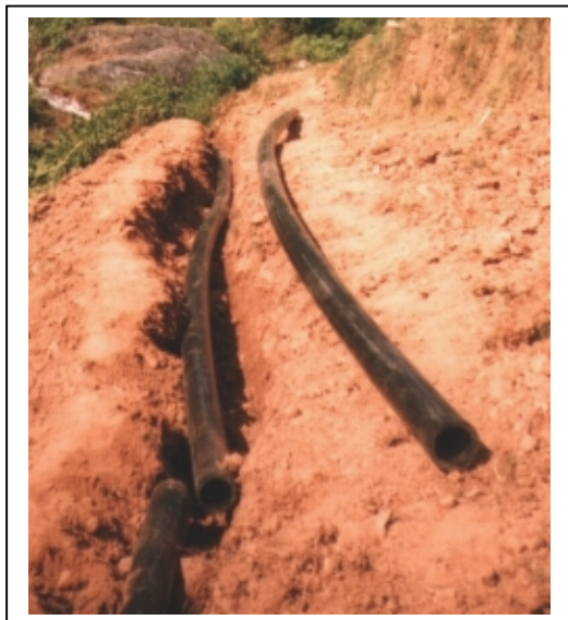
Figure 11-4 The penstock can be laid in a trench and then buried when the installation is complete to secure it
