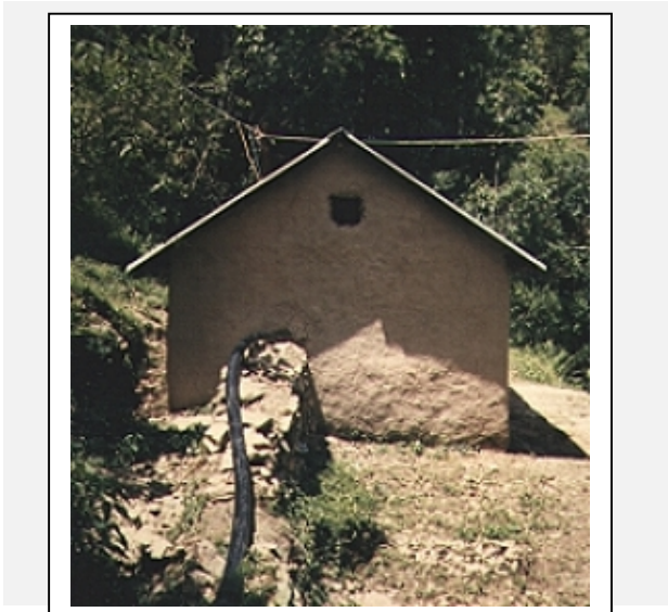
Figure 12-1 Typical stone powerhouse in Nepal
