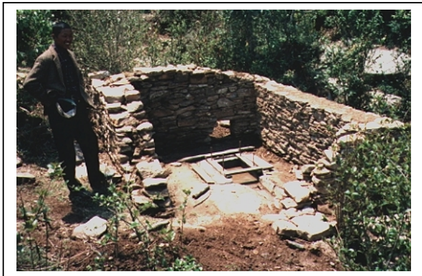
Figure 12-3 Power house under construction, Nepal
