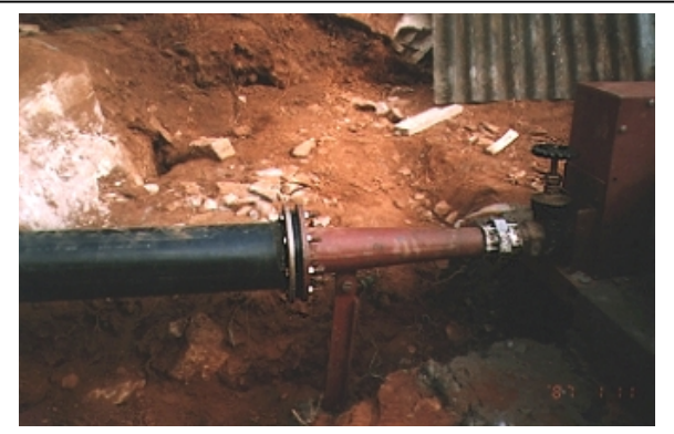
Figure 11-10 Penstock connection using flanges
