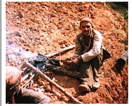
Figure 11-7 The metal plate is heated in a small fire
