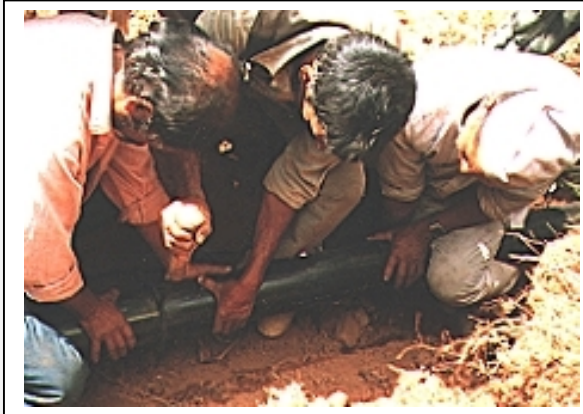
Figure 11-8 Both sides of the pipe are held against the hot plate.
