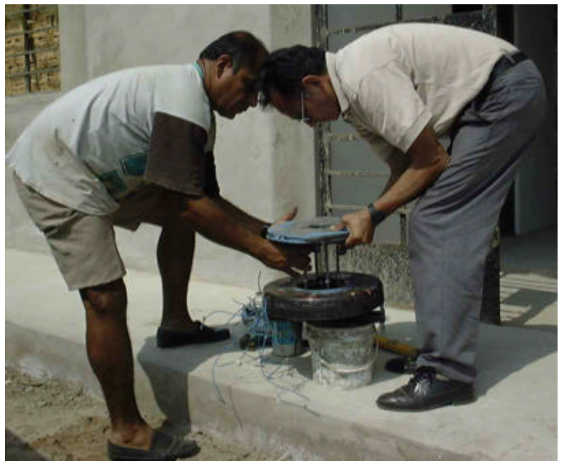
On site assembly in Peru
