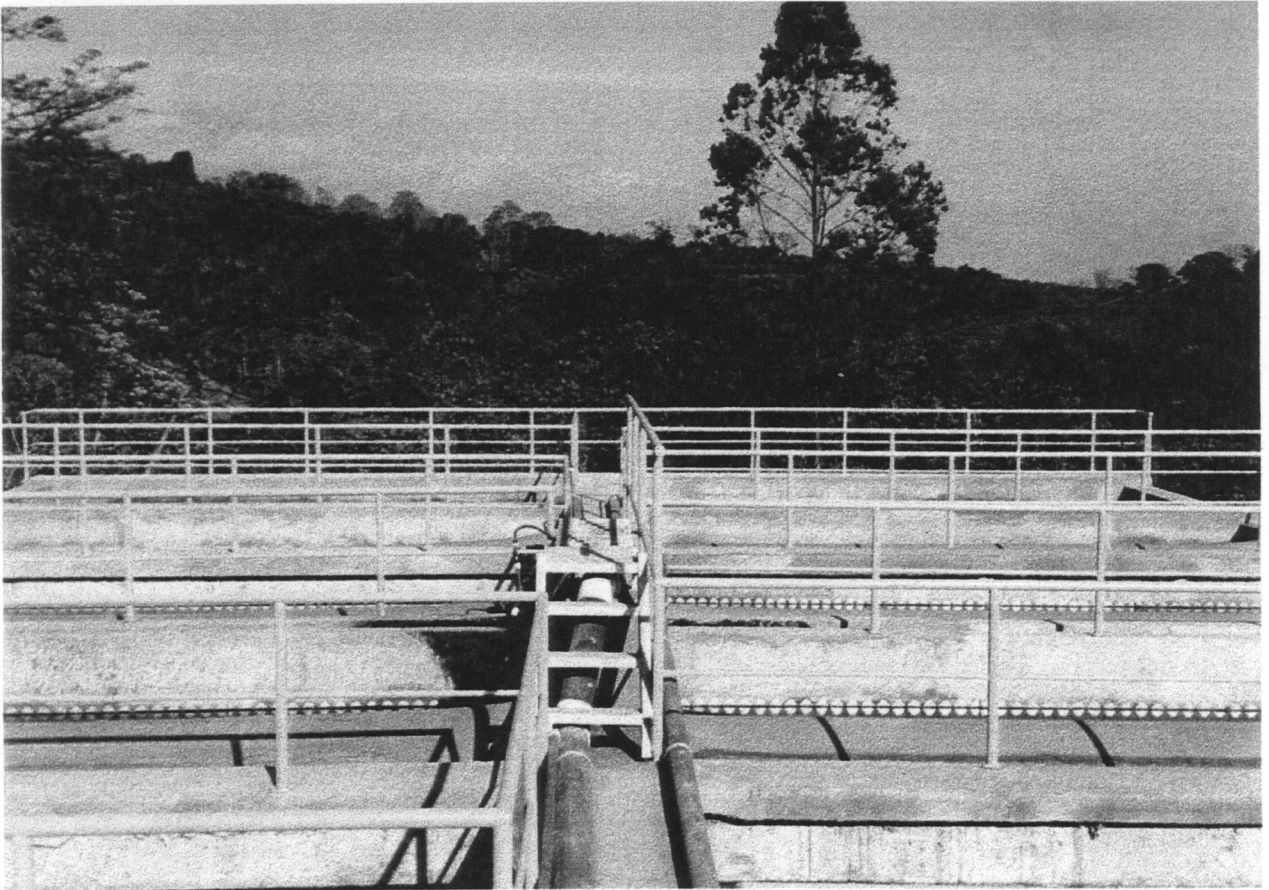
Naranjo Coffee Mill: Panoramic view of the anaerobic reactor
