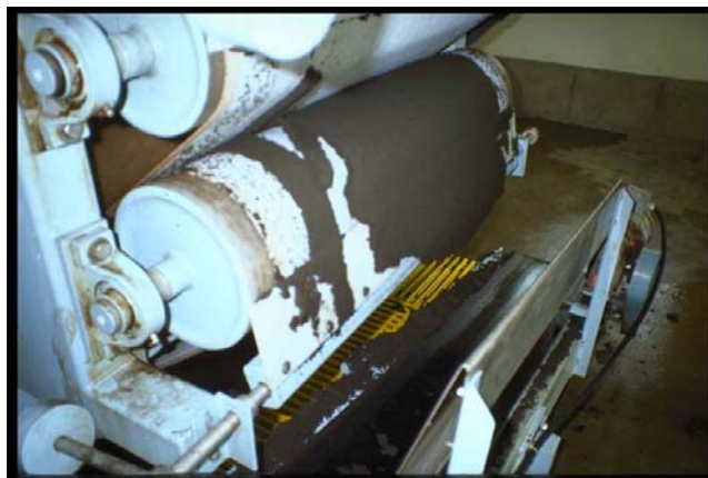
Figure 4.4 Picture of a belt filter 3
