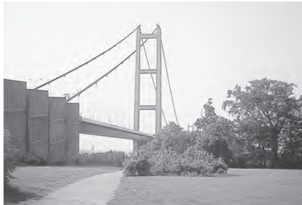
Plate 117 The largest structures in the landscape, such as the Humber Bridge, near Hull, UK, require plantations and tree clumps of generous size to maintain good generic scale relationships.
