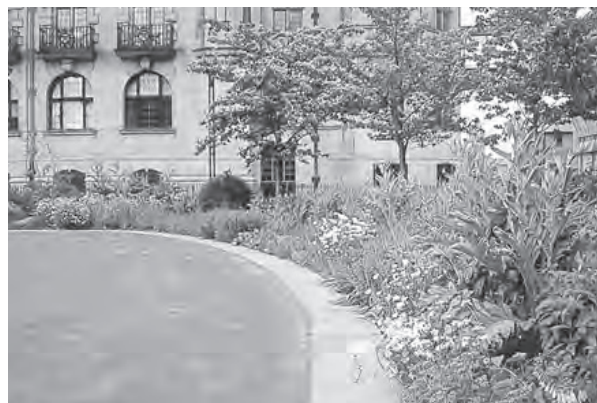
Plate 177 An edging of stone to a herbaceous border has many advantages. Grass cutting is easier, plants can be allowed to spread over the edge, access and work to the border in wet weather will cause less damage to the edge of the lawn, and crispness of line is visually satisfying (Sheffield, UK).
