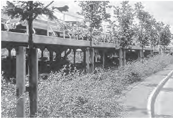
Plate 158 An urban hedgerow of Norway maple ( Acer platanoides ) planted in a hedge of Cotoneaster lacteus . The restricted width available for planting made this a suitable means of integrating the decked car park within the planting structure of the office development site.
