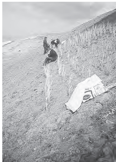
Plate 10 The indigenous European dune species, marram grass ( Ammophila arenaria ), is well adapted to this coastal fill site, but planting to assist establishment is necessary (Cumbria, UK).
