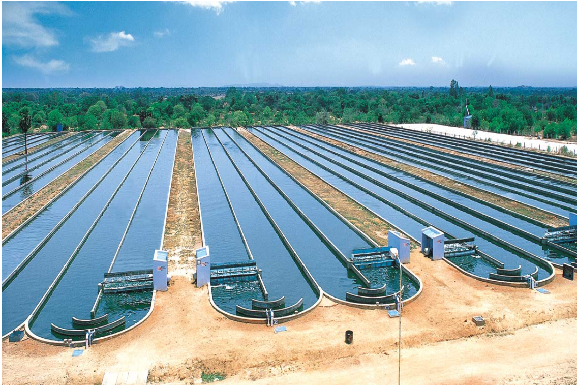
Figure 20. Spirulina raceway ponds, used by in India by Parry Nutraceuticals to grow Spirulina or Dunaliella .
