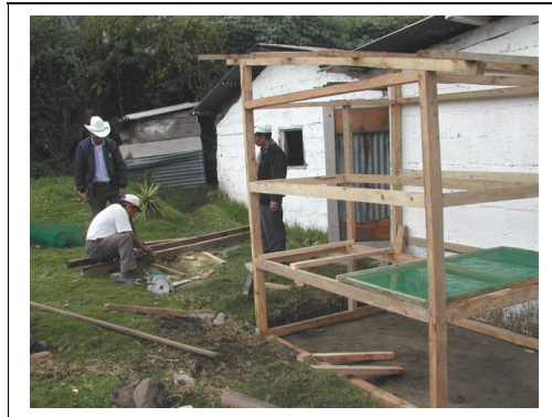
PHOTO 7: CONSTRUCTION D'UN SÉCHOIR, SIBINAL, GUATEMALA. [JDM, 2002]
