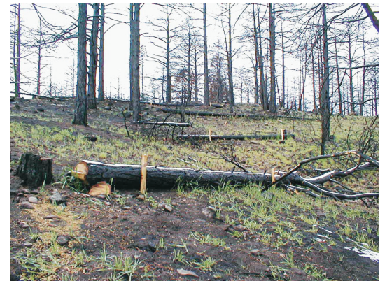
Contour log terraces (above and below).
