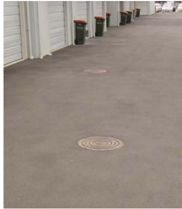
Photo 5 Rockbore Soakhole Installed beneath the pavement of a high density development
