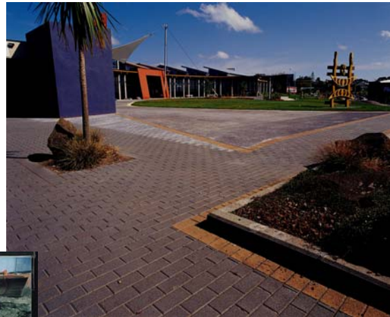
Photo 6 Porous Paving 80mm Enviropaver (photo supplied by Firth)
