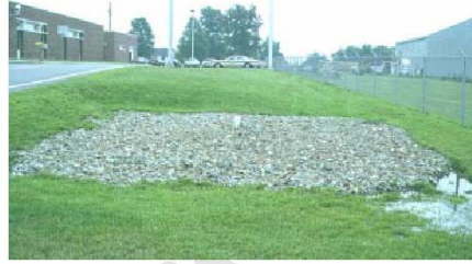
Photo 3 Filter-strip Soakhole (photo from ARC TP10 [3])
