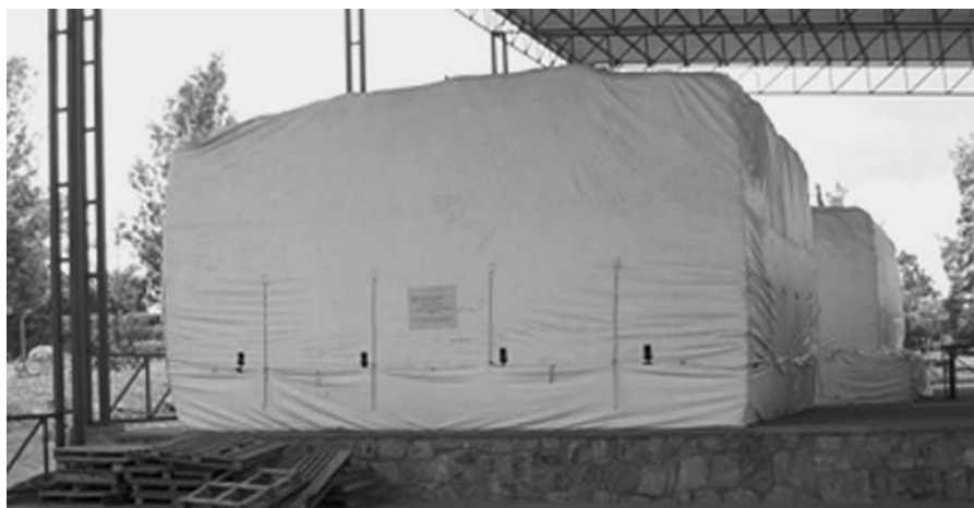
FIGURE 3.6. Hermetic grain-storage envelope sealed shut with a gastight zip in Rwanda
