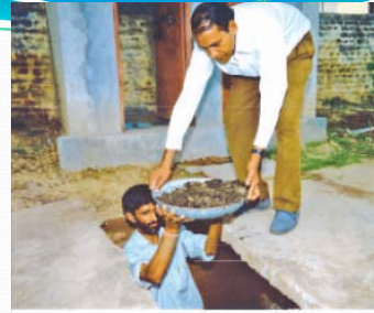
Taking out of manure from the pit of a Sulabh toilet
