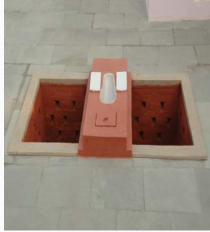
Sulabh pour-flush toilet for least space with toilet on top of pits
