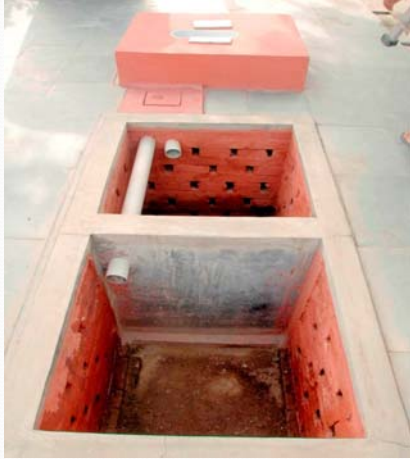
Sulabh pour-flush toilet for linear space with common dividing wall
