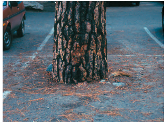
Figure 3.103. High risk of failure: Roots within CRR are more than 40 percent damaged, decayed, severed, or dead.
