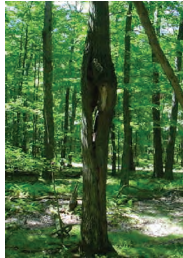
Figure 3.14. Bulges often indicate decay.
