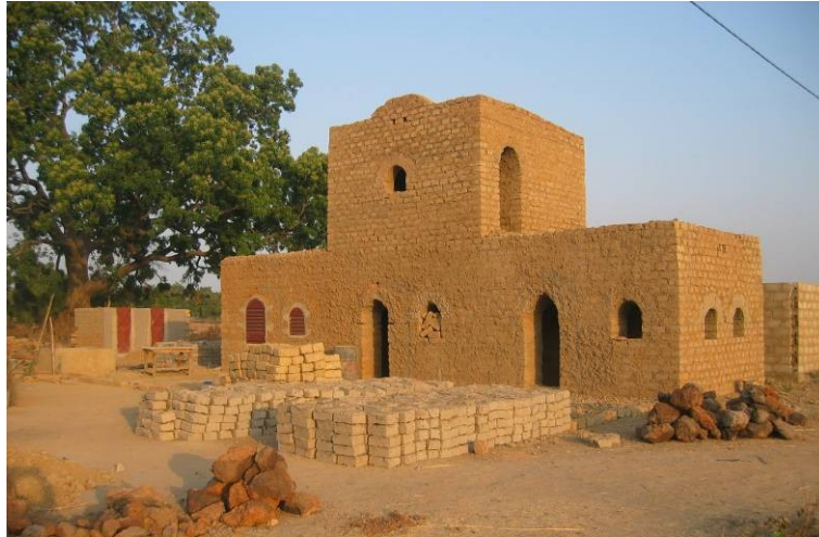
Figure 5 Two-storey house at Boromo, Burkina Faso
