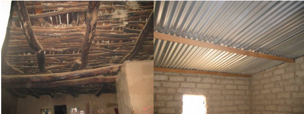
Figure 1: Traditional and 'modern' roofing in the Sahel
