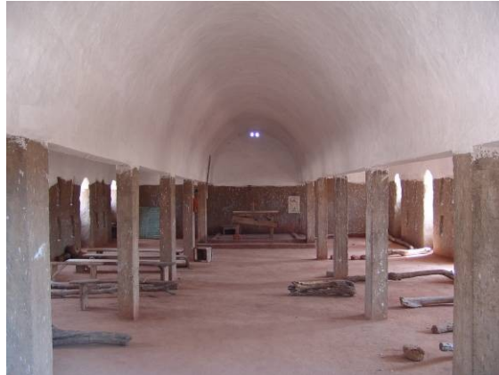
Figure 7: Church at Petit-Bale, Burkina Faso, with concrete beams and pillars supporting vaults
