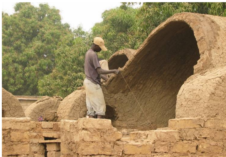
Figure 8: Vault construction using the guide cable
