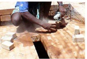
3. Grind a block to adjust its length
