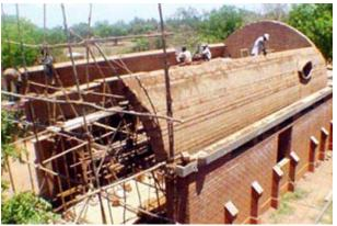
Building a semicircular vault of 6m span
