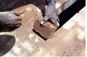
5. Insert the block. Note the mortar on the sides
