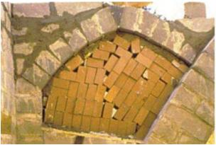
Masonry centring, ~ 80 cm span
