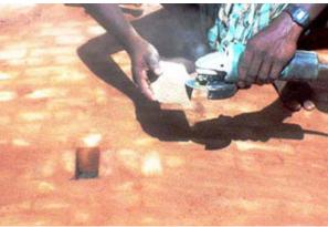
8. Grind the keystone to adjust its thickness
