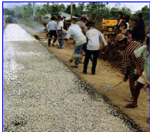
Image 4 – Hand Laid Bituminous Surface Dressing
