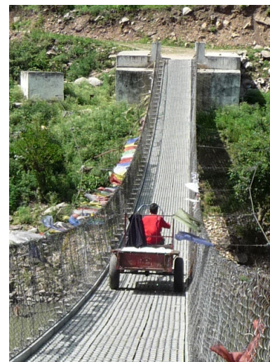
Power tiller bridge in Khoma
