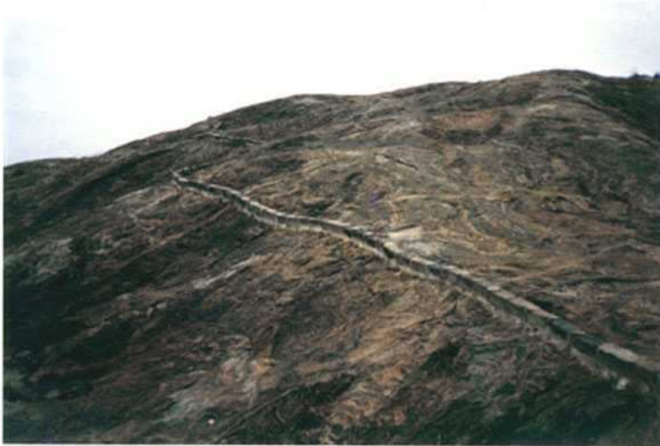
Plate 6.1 Water harvesting from a granite outcrop, Kenya. A stone wall about 20 cm high leads run-off to a storage dam out of picture to the right.
