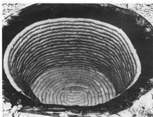
Plate 6.9 Two examples of the 'sausage' method of constructing water storage tanks (Intermediate Technology Development Group)
