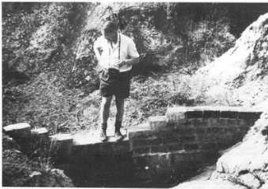
Plate 6.7 A simple sand trap weir, Zimbabwe
