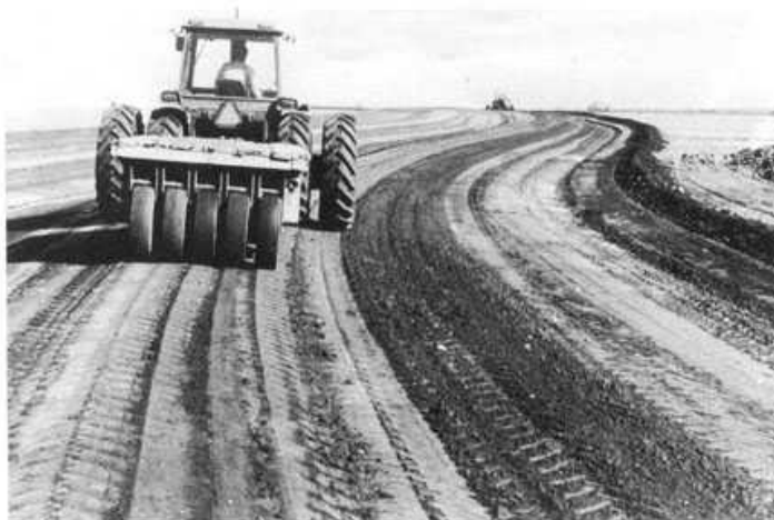
Plate 6.3 Smoothing and compacting the 'roads', Australia (I.A.F. Laing)
