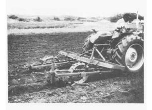
Plate 5.11 The ridger lifted by eccentric wheel (T.F. Shaxson)
