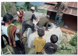
A rainwater storage tank constructed by householders in Nepal. (RAIN)
