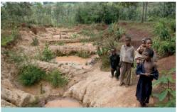
Check dam ponds for gully reclamation on gentle slopes and recharging of groundwater (HP. Liniger)
