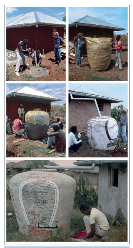
Steps for constructing a cement water tank using a plastic bag filled with straw. Drawing on tank shows design and material needed. (HP. Liniger)
