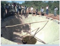
Cement-lined underground tank in construction, Ethiopia. (HP. Liniger)
