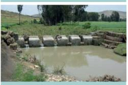
Check dam made of stone, concrete and gabion for irrigation purpose at the same time reducing the runoff velocity and enhancing gully rehabilitation. (E. Yazew)
