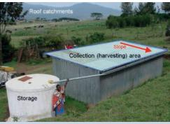
Roof catchment in Kenya showing the different components of a rooftop WH system. (M. Malesu).
