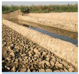
Water spreading weirs built in series (GIZ, 2011).
