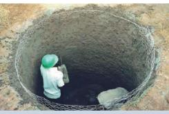
Underground tank for courtyard and road water harvesting, Kenya. This tank was equipped with a silt trap and used for storing runoff (Nissen-Petersen, 2007).
