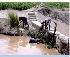
Blocking scour sluice on a modernised spate irrigation system in Yemen. (spate-irrigation.org)
