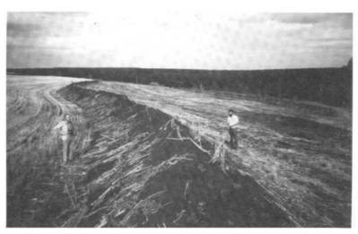
Plate 4.10 Murundum terrace in Brazil, intended to hold all surface run-off, even during heavy storms (T.F. Shaxson)
