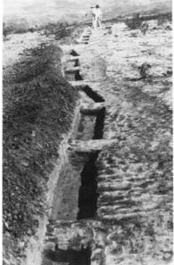
Plate 4.16 Hillside ditch with lock and spill drain (USDA)
