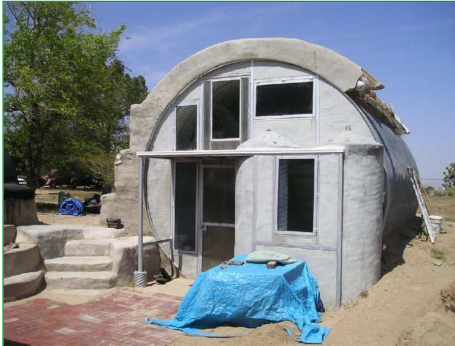
CalEarth Vault under construction. Photo by Ashley Muse www.flickr.com
