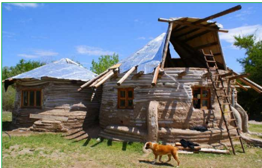
Earthbag Home under construction in Argentina. Lots more images here:
