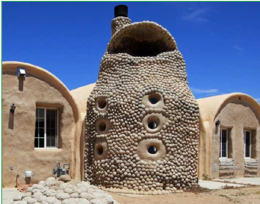
earthbag home Classical Arches, domes and vaults updated. The combination fireplace and wind-scoop faces prevailing winds. Photo by James flickr.com
