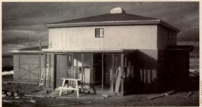
Straw-bale/adobe prototype home under construction (southwest elevation).
