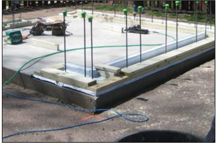
Figure 2: vertical reinforcing bars in foundation
