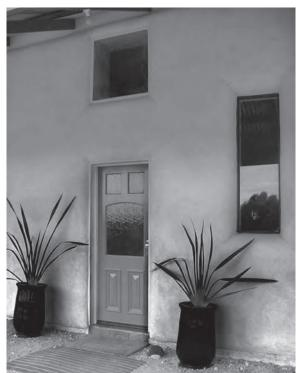
Figure 5.4 Completed door and window buck made from 190  $\times$  45 timber
