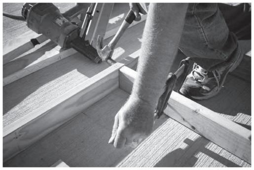
Figure 6.12 Fixing a twisted stud into a timber framed wall using a clamp to hold the stud in the correct position
