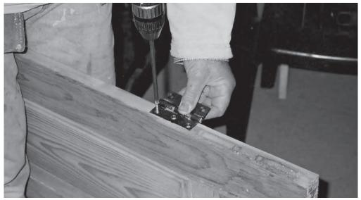
Figure 14.3 Fit the hinge to the door
