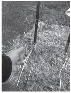
Figure 4.15 The twine is tied around the new length bales
