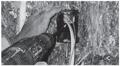
Figure 12.4 Screw the plastic electrical wall box to the timber peg
