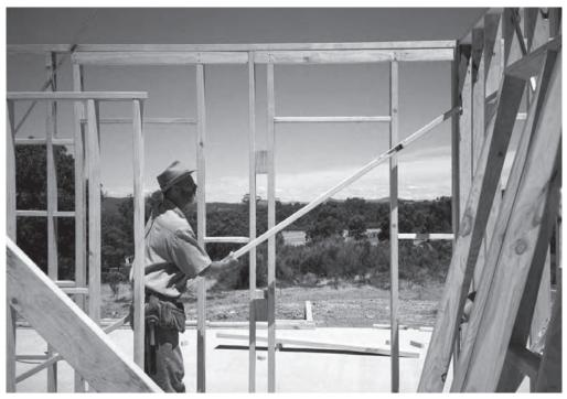
Figure 6.18 Force wall frames into a vertical position using  $90 \times 35$  pine
