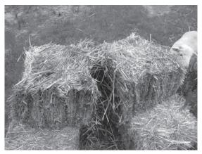
**Figure 4.16** The original ties on the bale are cut and the bale is separated into the two new lengths
