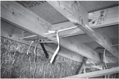
Figure 4.3 The intermediate securing of straw bales to the upper floor joists to prevent the 4.2 metre wall from toppling over during construction
