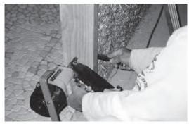
Figure 14.9 Fix the bottom of the jamb stile to the frame
