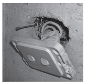
Figure 12.5 Render over a metal mounting plate with a plastic shroud at its rear
