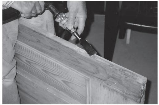
Figure 14.2 Make a checkout in the side of the door for the hinge
