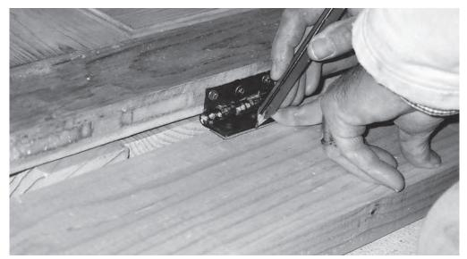
Figure 14.4 With the hinge fixed to the door, mark the door jamb stile
