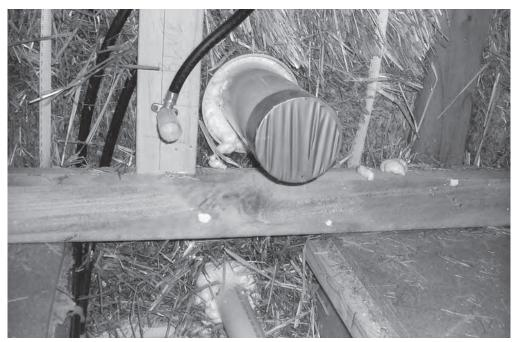
Figure 13.1 100 mm sewer pipe through 150 mm pipe with expanding foam sealant
