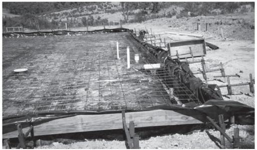
Figure 3.12 Plastic membrane and steel mesh supported on bar chairs for a concrete slab
