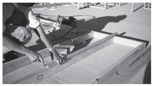
Figure 6.14 Marking the studs for the location of noggings using a nog marking stick
