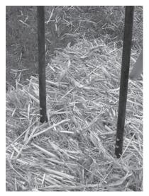
Figure 4.13 The double bale needle is inserted into the straw leaving the eyes of the needle exposed
