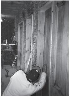
Figure 14.10 Check that the door and stile are parallel
