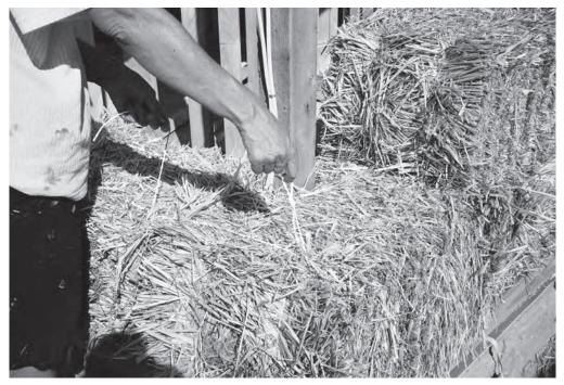
Figure 4.4 The corner bales are secured by tying the bales together with twine in two places
