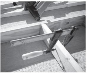
Figure 6.11 Use a clamp to straighten twisted studs prior to installation
