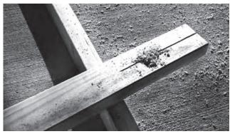
Figure 6.10 Rip cut in the end of a door opening stud in preparation for inserting a lintel
