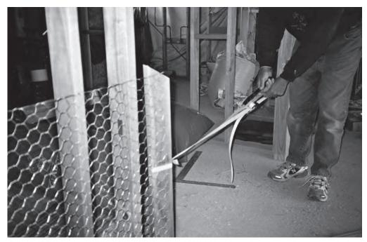
Figure 6.20 Tightening the wire netting across the face of the wall using the compression strap tensioning tool
