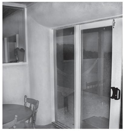
Figure 5.21 Completed render over the wire netting frame work at the stile of the door buck and door
