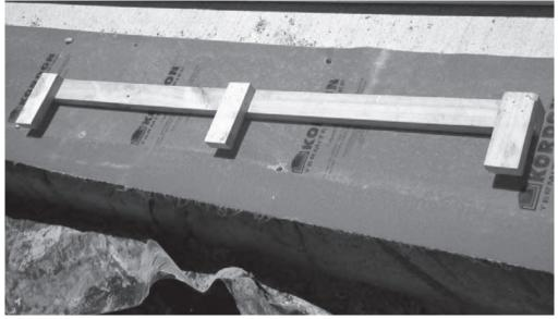
Figure 6.9 Gauge marker for marking the positions of common studs
