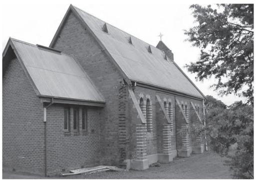
Figure 8.9 A church in Bendigo, Victoria, with buttresses that appear like wings along the outside of the walls to resist the outward pressure of the roof from spreading the walls
