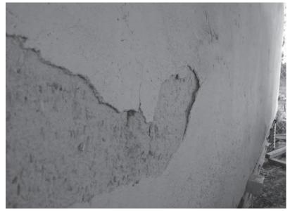
Figure 11.1 Delaminating of the third coat of render due to incorrect preparation
