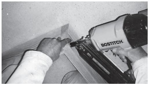
Figure 14.8 Fix the head of the door jamb to the stiles
