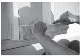
Figure 6.15 Marking the stud with the depth of the lintel to be fitted
