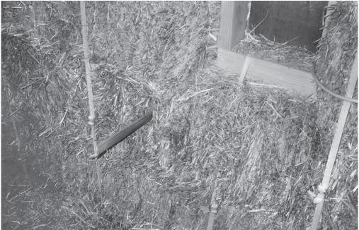
Figure 4.10 Markers are positioned in the straw bale wall as a guide for shaping the bales prior to rendering
