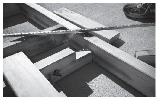
Figure 6.16 Completed checkout in the stud ready for the installation of the lintel
