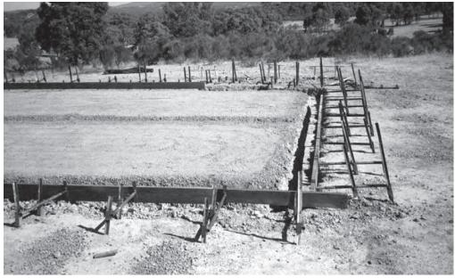
Figure 3.11 Compacted crushed rock and formwork for a concrete slab
