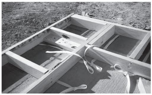
Figure 4.2 The bottom boxing to support a straw bale wall
