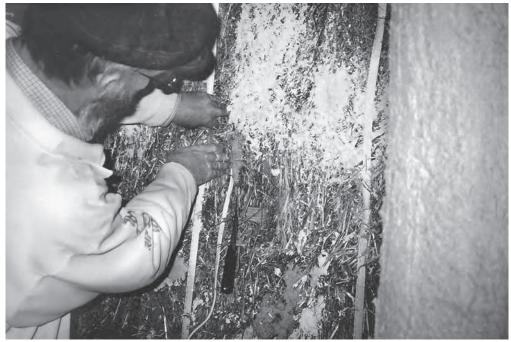
Figure 12.1 Cutting a slit in the straw into which the electrical cable is inserted
