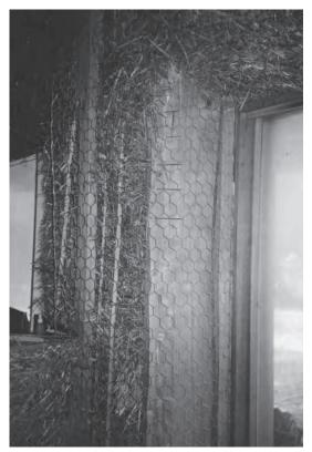
Figure 5.20 Wire over 290  $\times$  45 door buck stile to facilitate rounded render at the door opening
