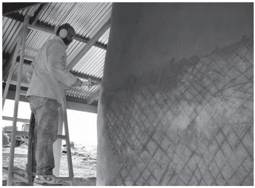
Figure 11.2 Scoring (hatching) of the second coat of render provides a fixing key for the next coat of render
