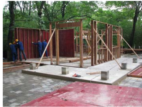
Figure 1: Installation of modular wall panels
