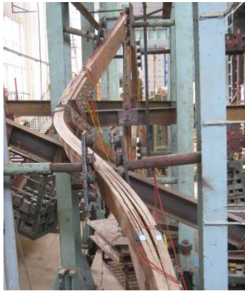
Figure 14: Failure of glulam truss
