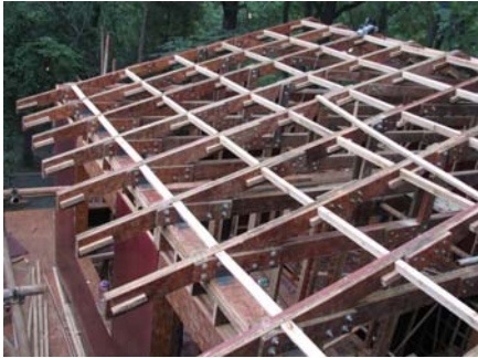
Figure 4: Installation of roof trusses
