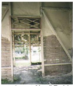
A few damaging house gave us solid proof of the bamboo mat as inner part of the wall. The skeleton could only be seen from the interior. They used mortar plaster by mixing sand with lime.
