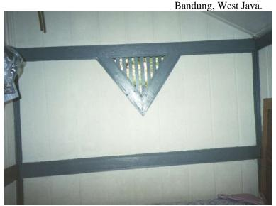
The walls made of precast panel have wooden skeleton. The lines between panels can not be seen clearly because covered by annually lime coat. This original house was the only left.
