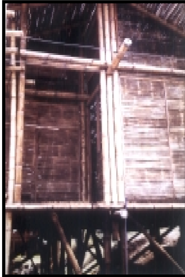
Fig. 94: A wall made of esterilla (Costa Rica)
