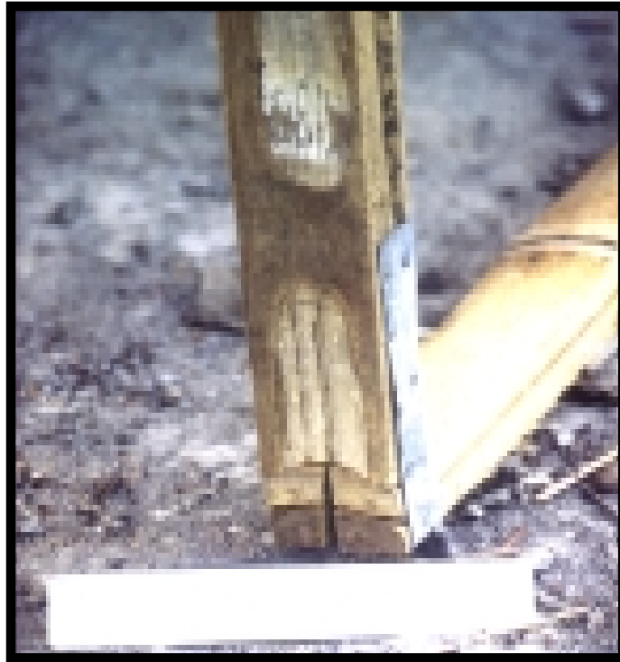
Fig. 69: Joint for the lower corner of doorframes
