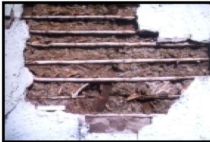
Fig. 96: A close-up of the solid bahareque wall (the plaster is missing) showing the basic technique
