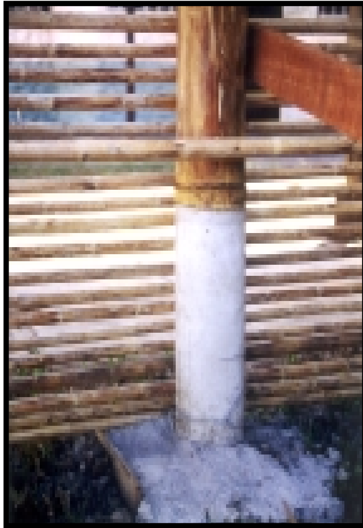
Fig. 18: Prefab concrete foundation for bamboo column
