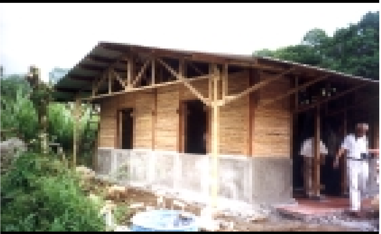
Fig. 92: A well-protected outside wall
