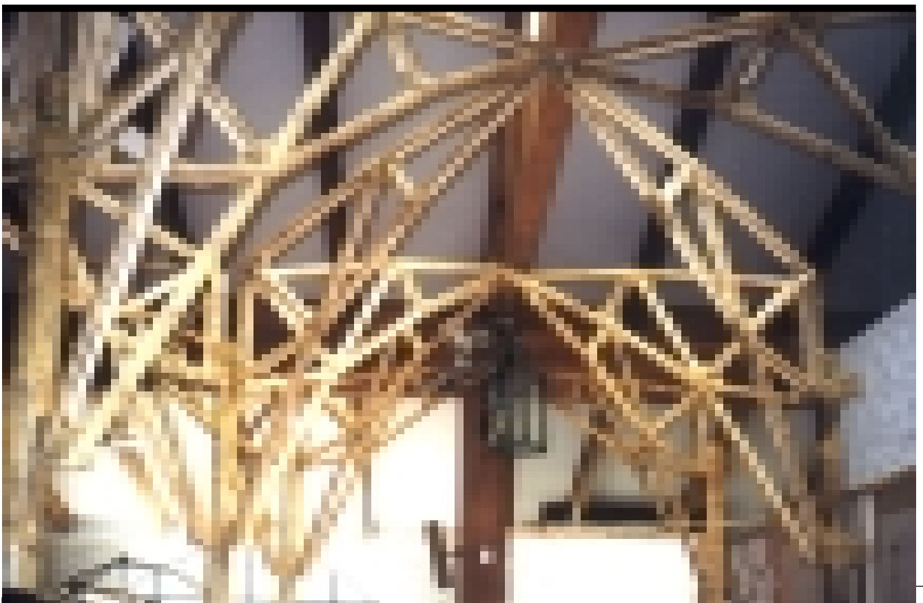
Fig. 72: Trusses in an exhibition area
