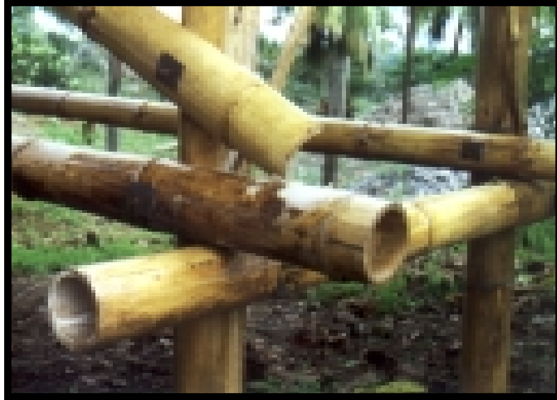
Fig. 64: A joint in Group 5, with steel bolts
