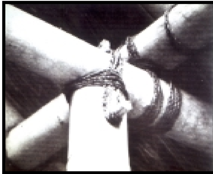
Fig. 61: A joint of the type 4.5 (Dunkelberg 1985)
