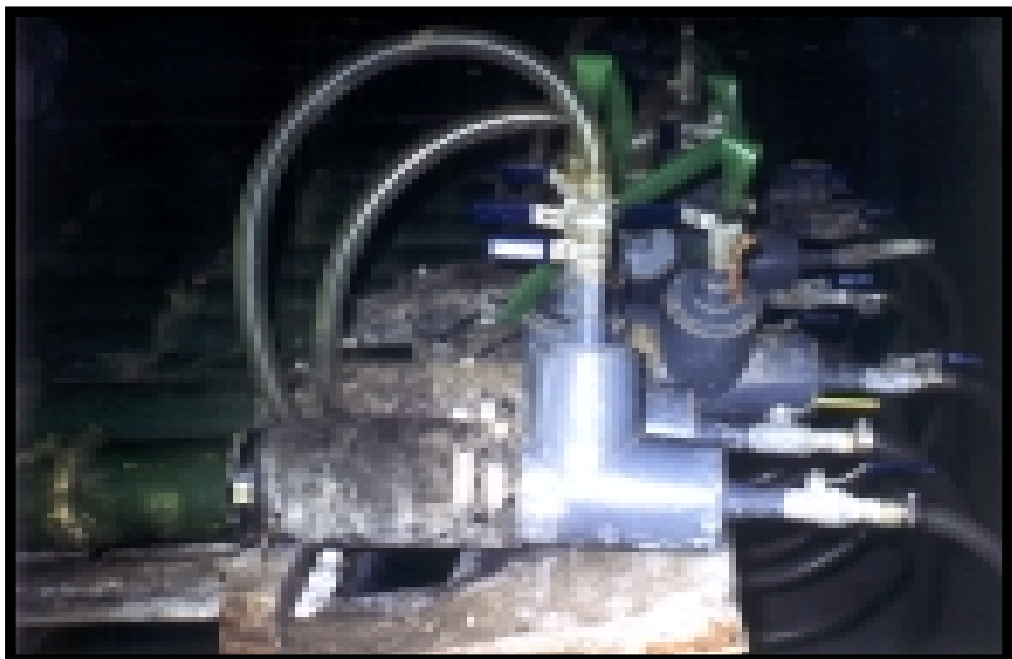
Fig. 39: Modified Boucherie treatment in progress
