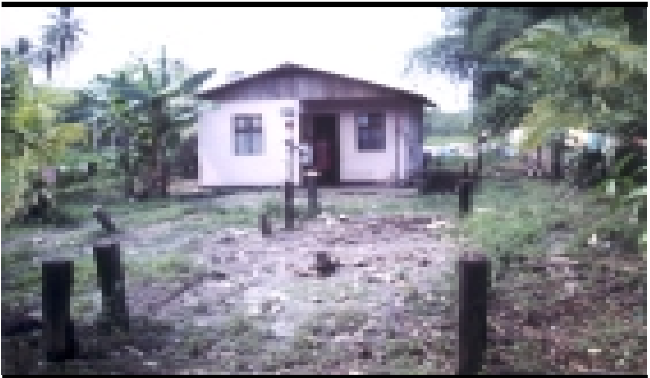
Fig. 90: A bamboo house that emerged unscathed from the 1991 earthquake (Costa Rica)
