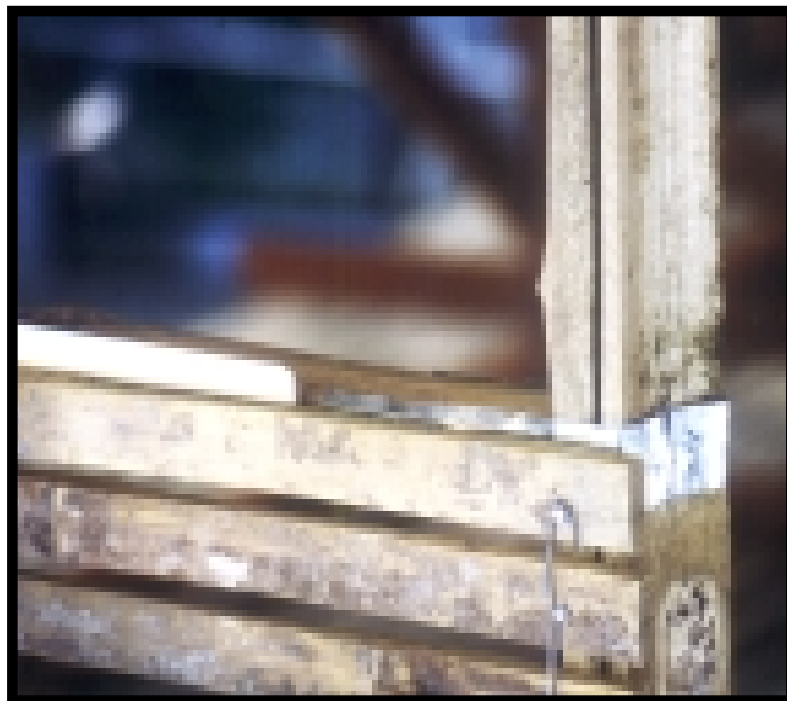
Fig. 70: Joint for the upper corner of doorframes
