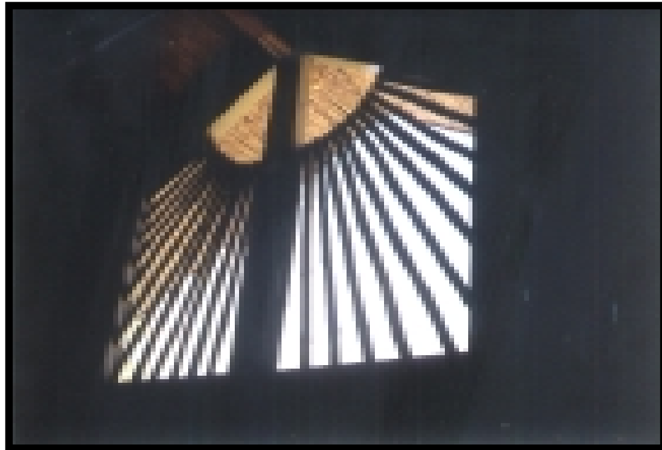
Fig. 98: A bamboo window
