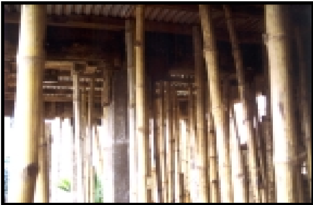
Fig. 84: Bamboo culms support concrete floor (Bangladesh)
