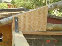
Pictures 25-26: Truss hanging and fixing
