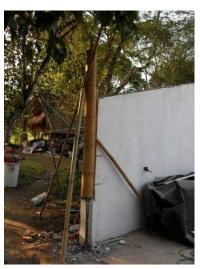
Figure 3: Bamboo Column establishment
