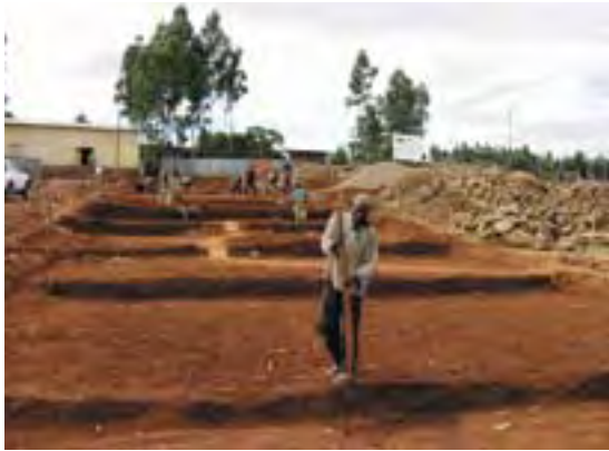
Levelling for the foundation is made
