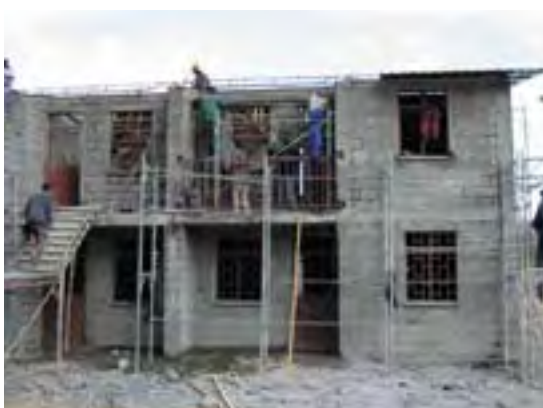
Starting the roof construction, street side view
