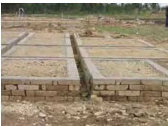
The finished foundation
