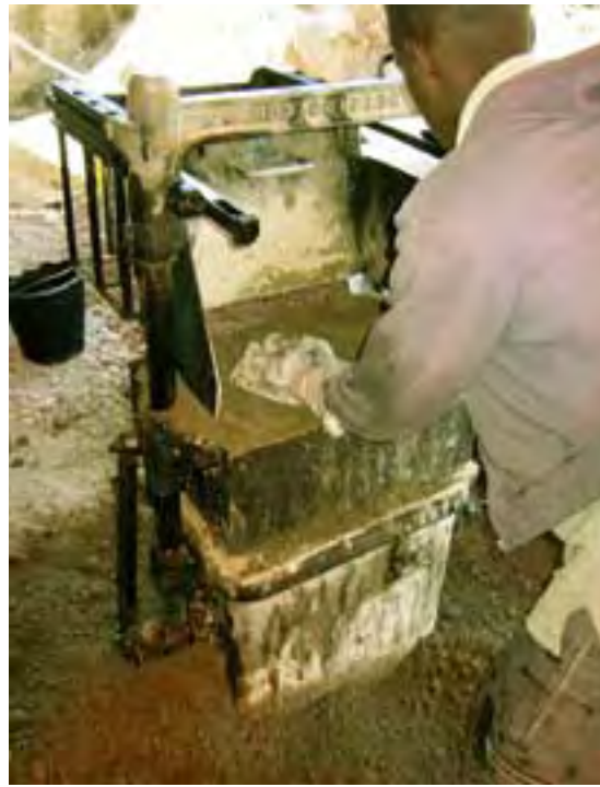
Concrete is filled up during compacting until the molde is filled
