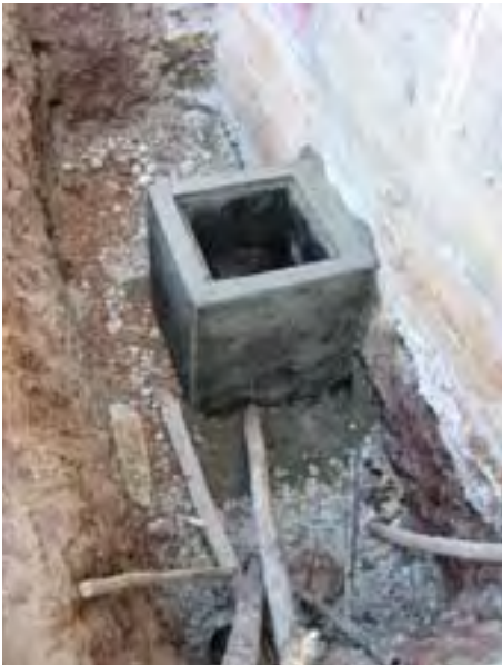
The pit for the manhole
