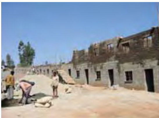
Finishing the upper floor, backyard view
