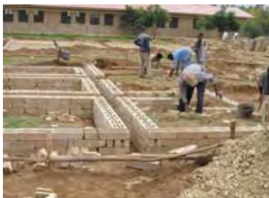
Lost formwork for foundation
