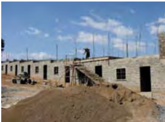
Ground floor finished, reinforcement for further walling, backyard view
