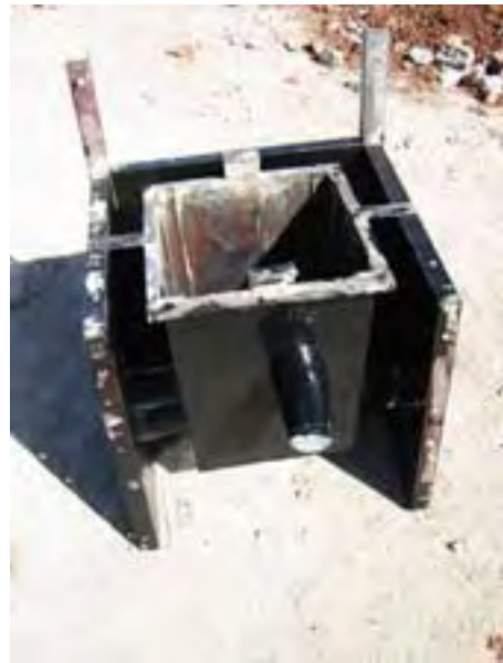
Formwork for the manhole, viewed from the side of intake (front panel removed)
