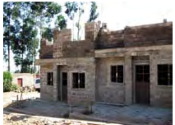
Starting the upper floor, street side view
