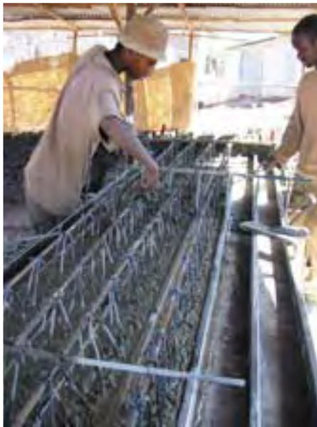
Filling in concrete by hand
