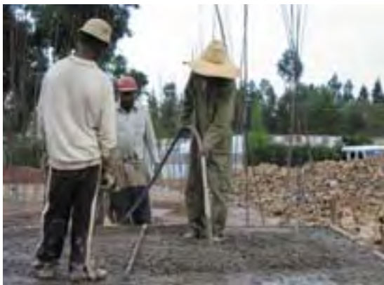
Construction of foundation using compactor
