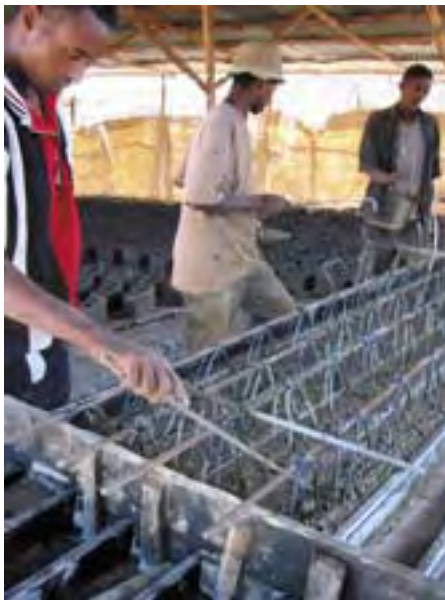
Spreading the concrete, using a bend bar
