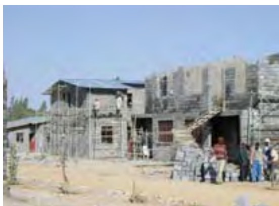
Starting first floor
