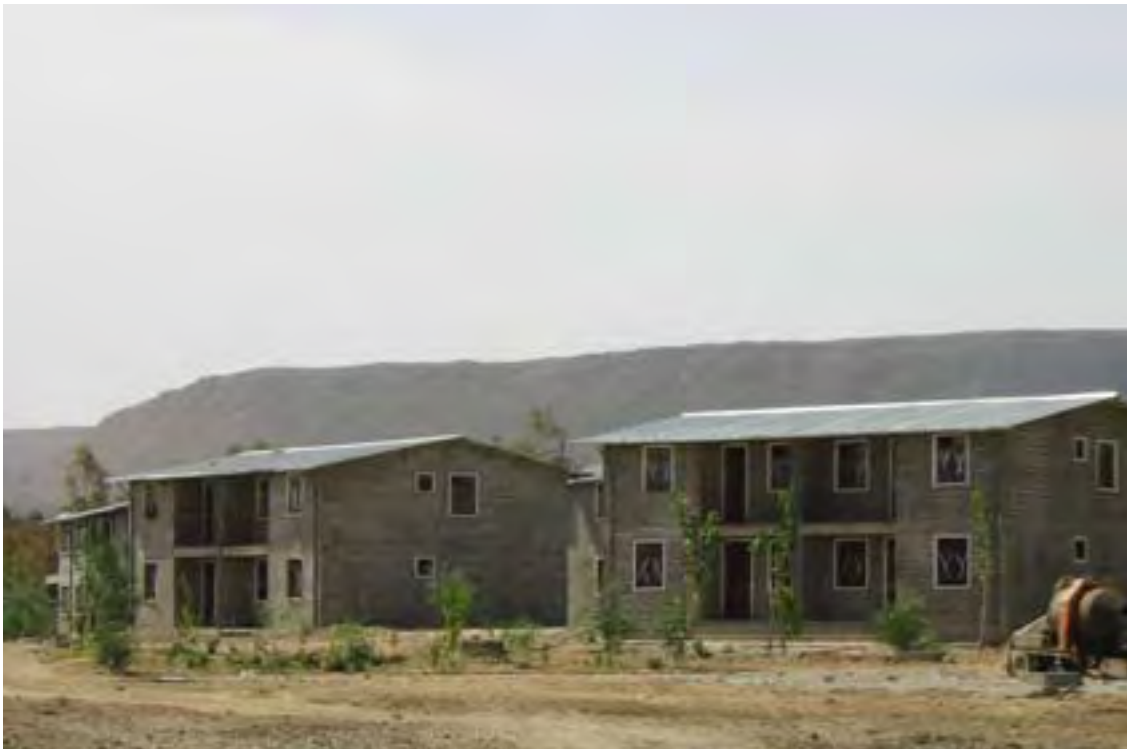
Settlement area in Mekelle
