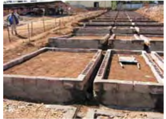
Preparation for combined strip and mat foundation
