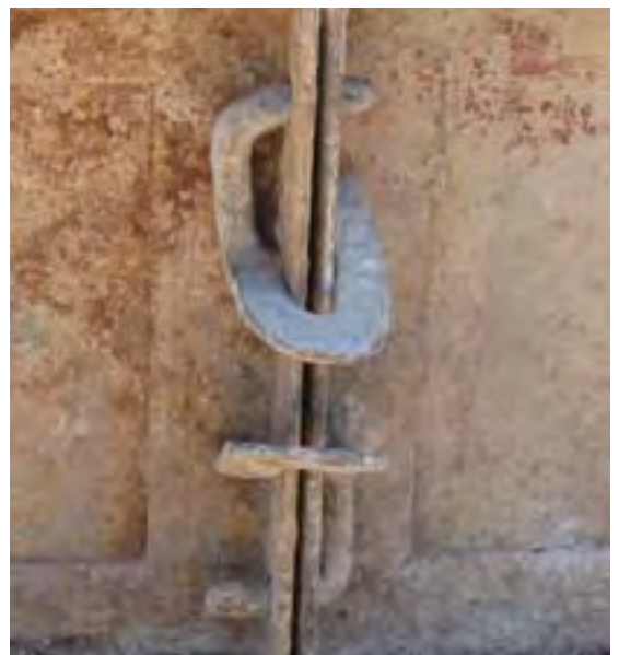
Two clamps mounted on formwork for foundation
