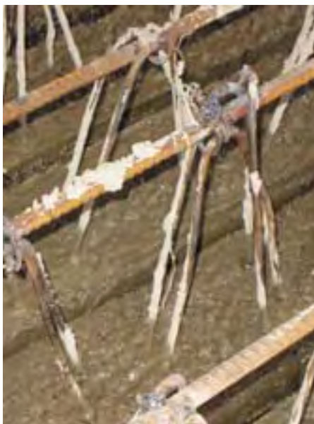
The precast-beams after removing the mould
