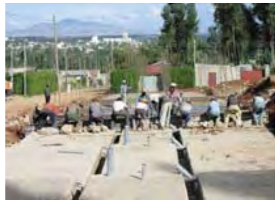
Sanitary pipes are installed
