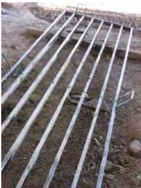
Mould for the pre-cast beams
