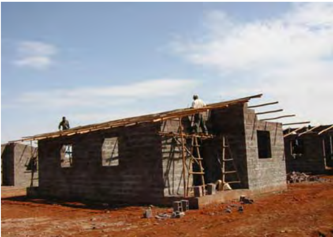
Construction of Houses in Bahir Dar
