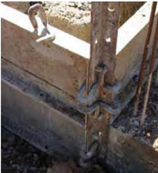
The edge of a formwork-assembly for foundation
