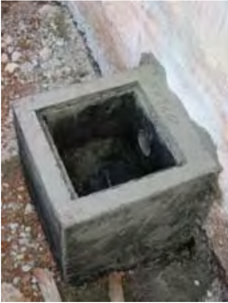
The cast manhole
