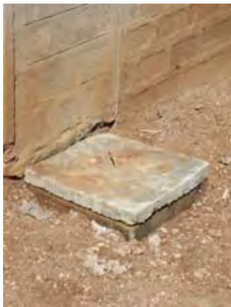
The manhole covered with a precast lid
