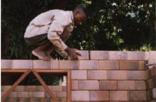
Foundations are made using the same blocks reinforced with mortar, building then commences above by dry stacking the blocks one on top of the other.
