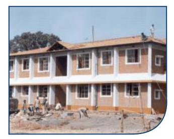
The LCH Technology allows "dry construction", i.e. no mortar is required to hold the bricks together. Made from soil treated with the RoadPacker C.B.S. product, the RoadPacker SEB's can be used almost immediately, after curing. The fast, reliable and easy to handle, SEB machine, will allow for low cost construction of high quality houses with unskilled labour.
