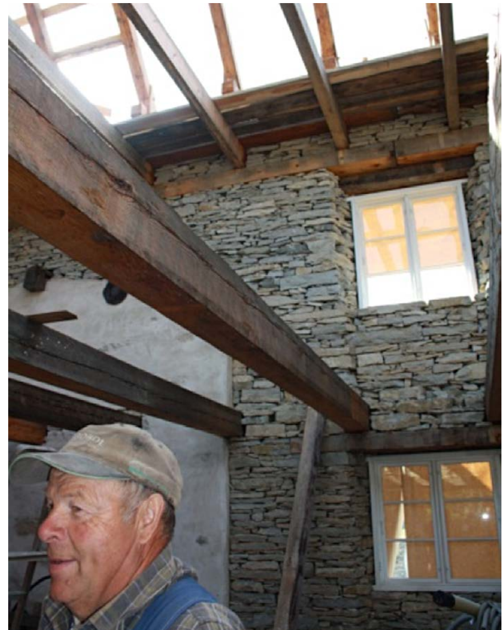
Figure 10. The interior of a new two-storey house which is being built without mortar. Its builder, master mason Erik Larsson to the left. Photograph by Anna Plahn.
