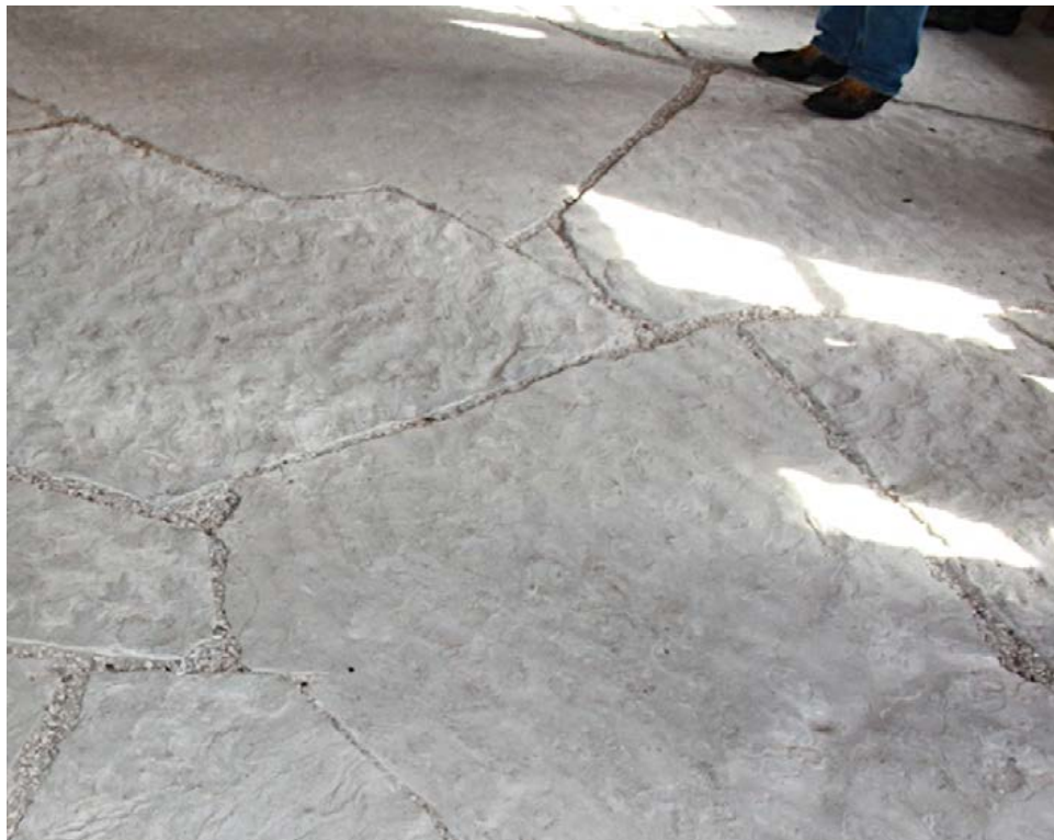
Figure 9. Floor of very big flagstones of Gotlandic limestone. Photograph by Anna Plahn.
