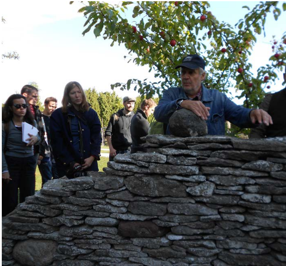
Figure 12. When you take a longer brake from building you can make the working joint invisible by making it at an angle. Stefan Haase (in the middle) instructing students. Photograph by Kirsti Horn.
