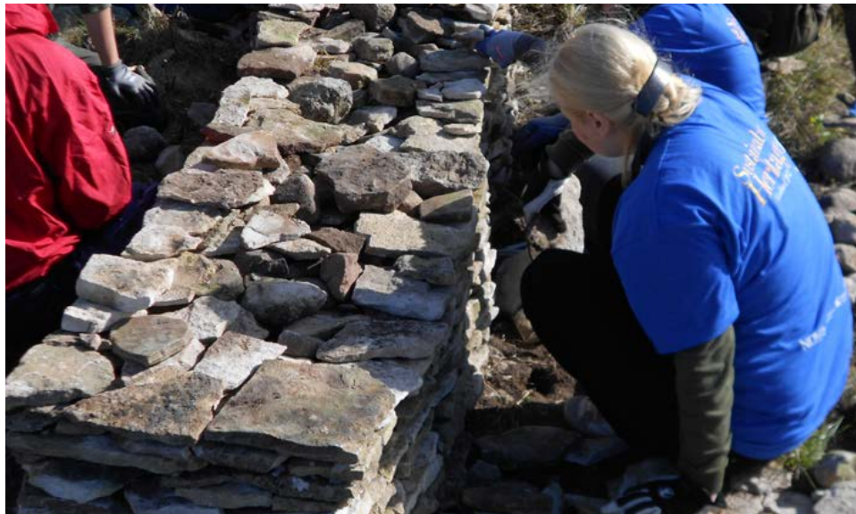
Figure 19. Student experiments: lime stone wall being constructed. Photograph by Kirsti Horn.
