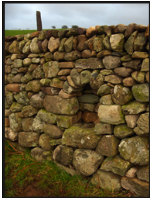
An arched niche incorporated into a farm wall built by Sean.
