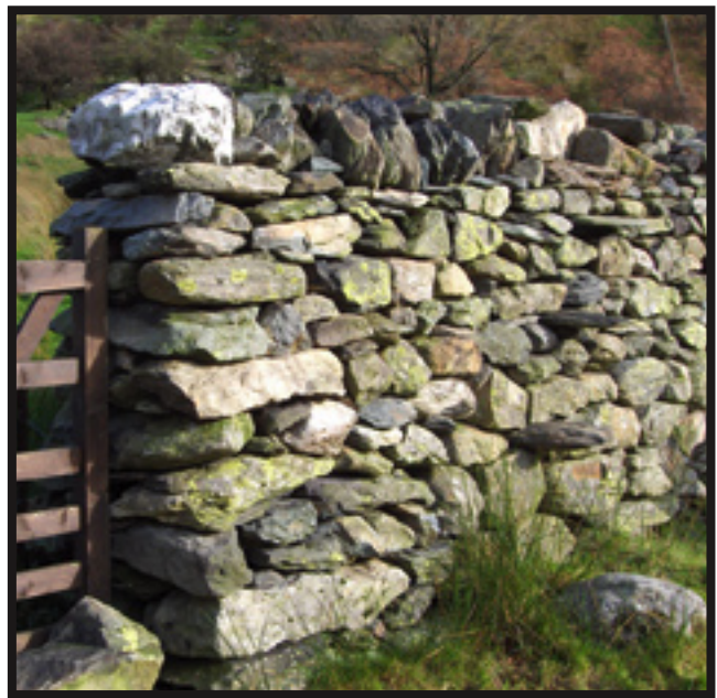
A well built wall end of fairly irregular stone.
