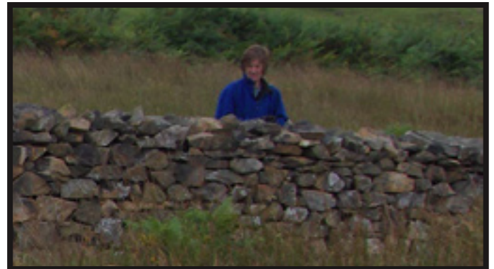
Vanessa putting the finishing touches on a section of wall
