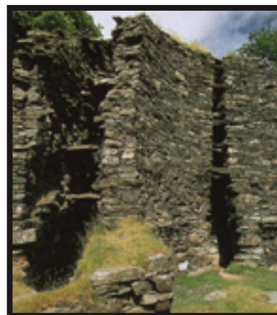
Dun Troddan, one of the brochs of Glenelg, shows the hollow wall construction. (Photo: Noonan, 2000)
