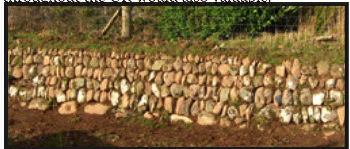
A newly repaired Welsh Cawdd.
