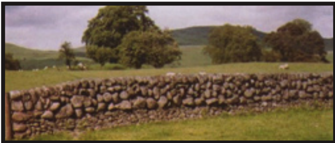
A galloway dyke. In this wall the double section comes only a third of the way up the wall. (Photo: Dry Stone Walling, Techniques and Traditions, 2004)
