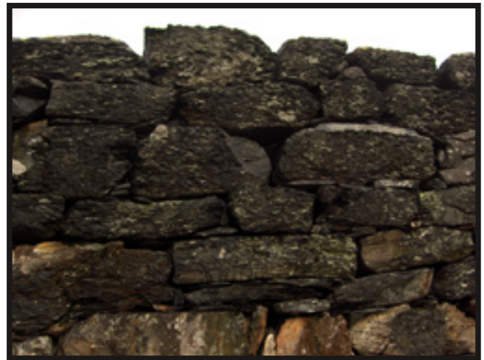
Looking up at the face of the wall.
