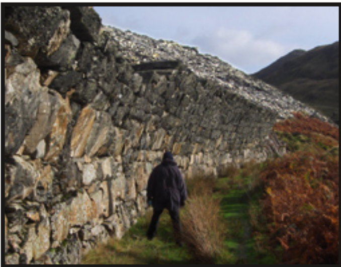
Looking along the wall from below.
