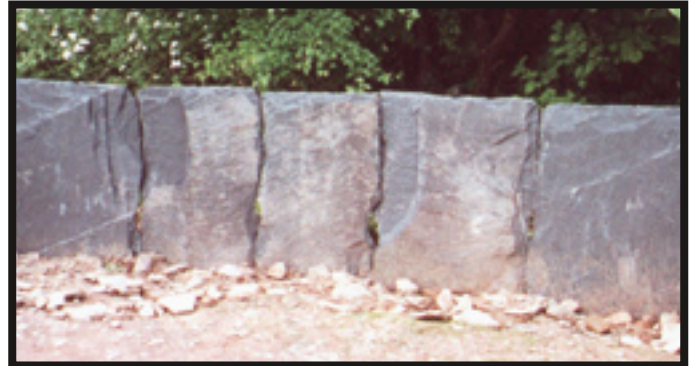
A slate fence made of slabs in the Hawkshead style with the slabs interlocking. (Photo: Dry Stone Walls, the National Collection 2002)
