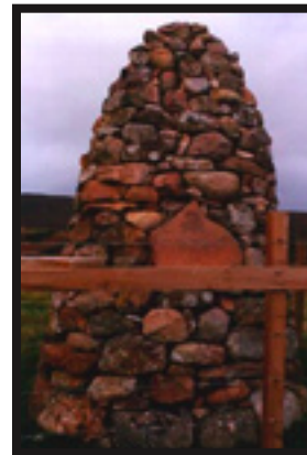
A dry stone cairn monument. Note: the fence in front is not part of the cairn. (Photo: DSWA Picture Gallery, 2005)
