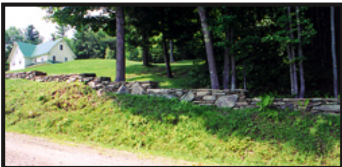
A wall built during the summer of 2003
