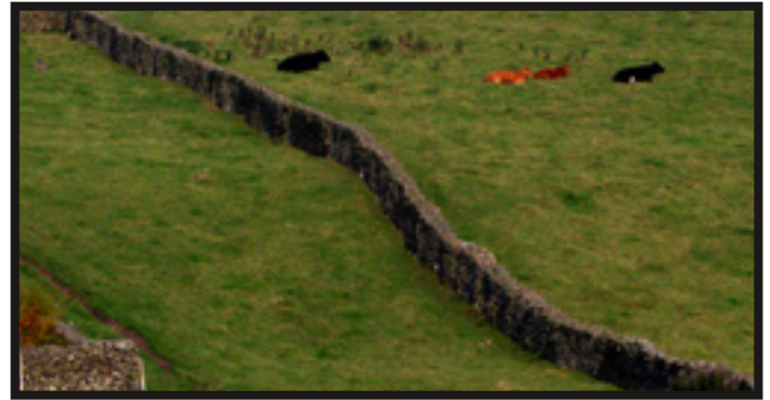
This old farm wall has an uneven batter which results in a blochy shadow pattern.
