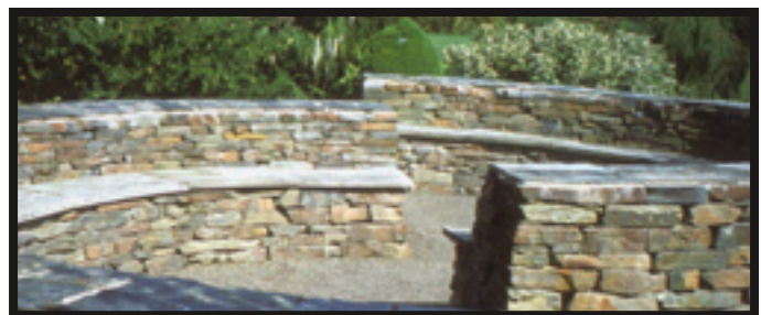
A seat wall with flat cap stones. In this case the cap stones were mortared, but this is generally not necessary. (Photo: Garner 2005)
