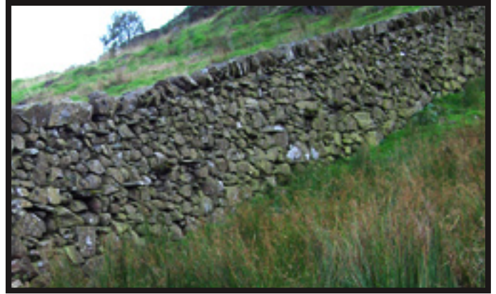
A fine section of Lake District wall running up a steep slope. Note the though stones are a constant height above the ground.
