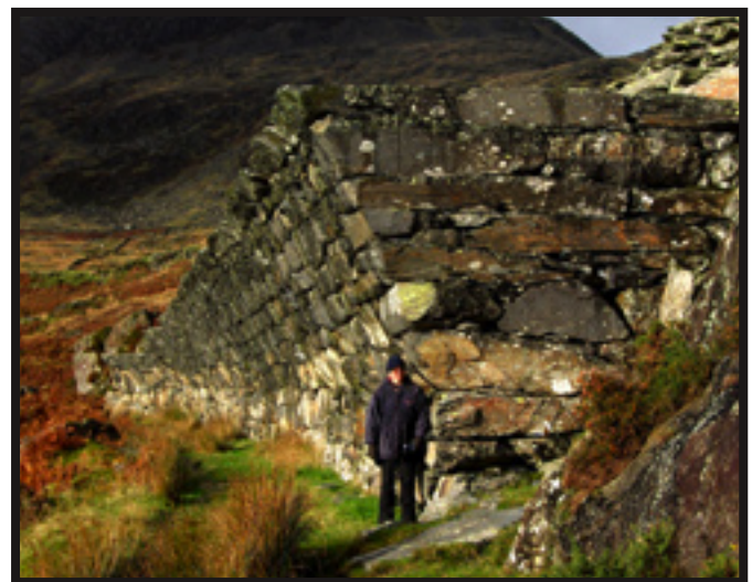
Looking at the top end of the wall. Note the length of the stones used to achieve the overhang.
