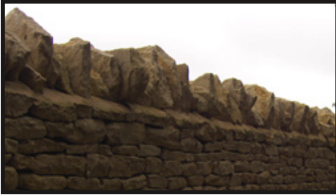
A new roadside wall with a mortared cope.
