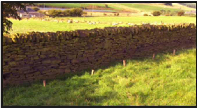
An old field wall built of level bedded sand stone.
