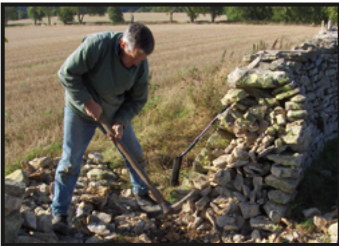
Andy stripping out an old field wall.
