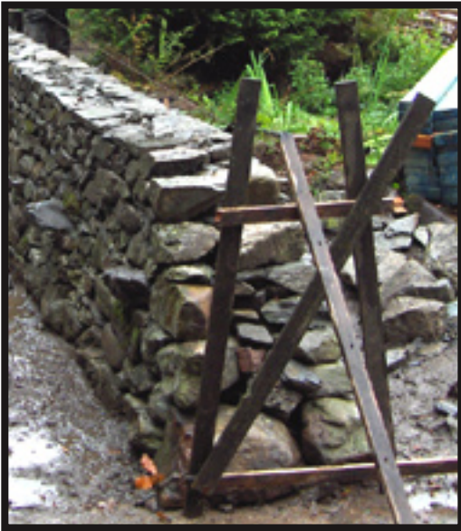
A bater fram in use. Once the wall is built up to the frame, as in this picture, the frame is then moved back, and another section of wall is built
