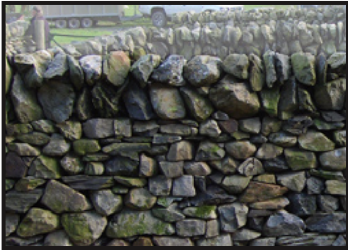
A wall with a double cope.
