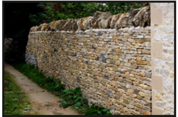
A tall freestanding wall built by Andy.
