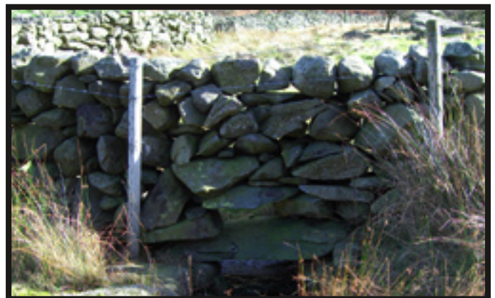
A single wall bridging a stream.
