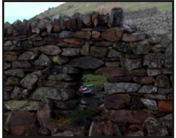
A lunky built by the author under the supervision of Sean Adcock.
