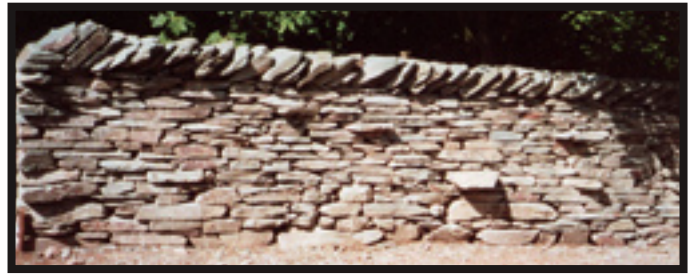
A wall with the stones kept level throughout. (Photo: Dry Stone Walls: The National Collection, 2002)
