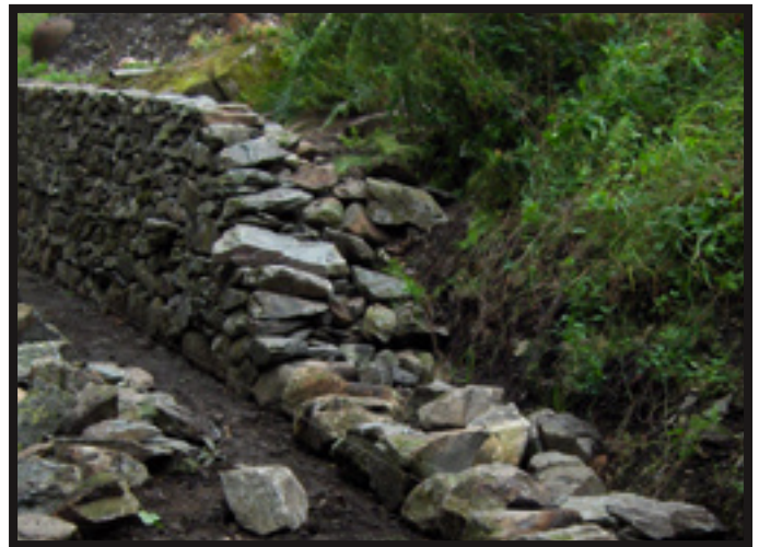
Building a single faced retaining wall.
