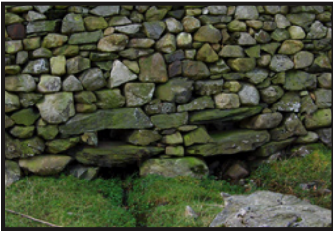
A double water drain with two gaps in each.
