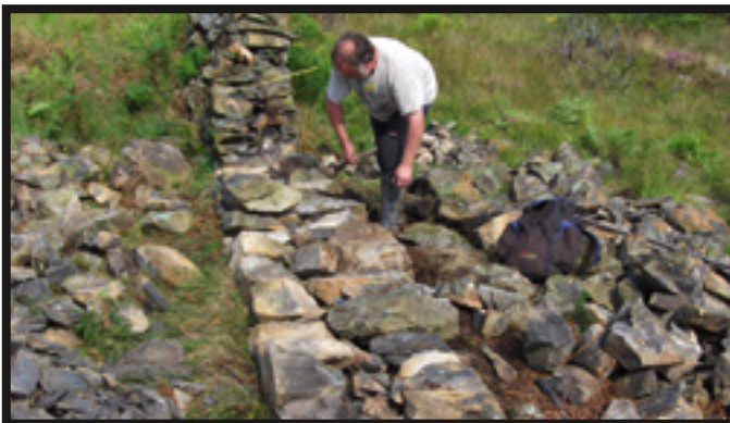
Jerry at work building a wall.
