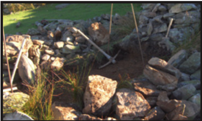
A section wall stripped out and ready for rebuilding.
