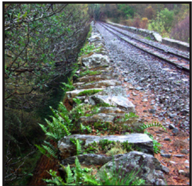
Looking down the north face of the wall.
