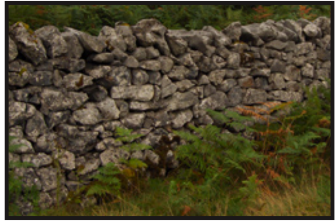
A Lake District wall, not yet fall, but in need of rebuilding.
