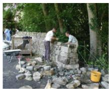
Fig. 8 Rebuilding a section of dry stone wall – note the construction of the wall-head.
