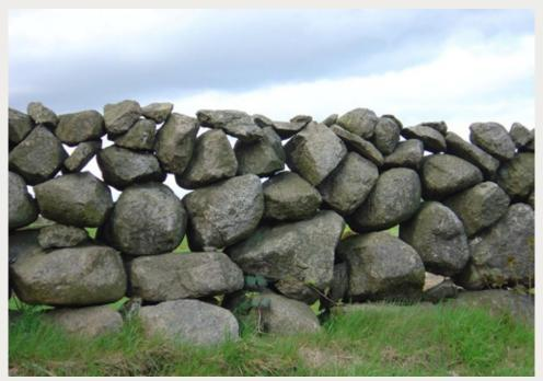
Fig. 3 Single wall or boulder dyke.
