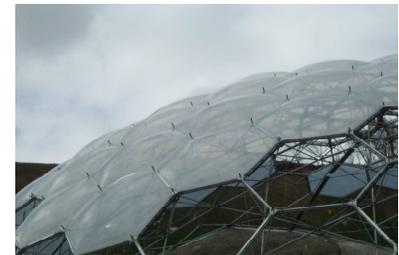
1.13 Specially designed connectors were designed to connect the ETFE pillow membranes to the steel structure.
