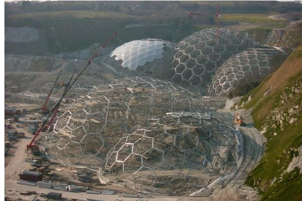
1.07 The domes under construction against one of the side walls of the old clay quarry.
