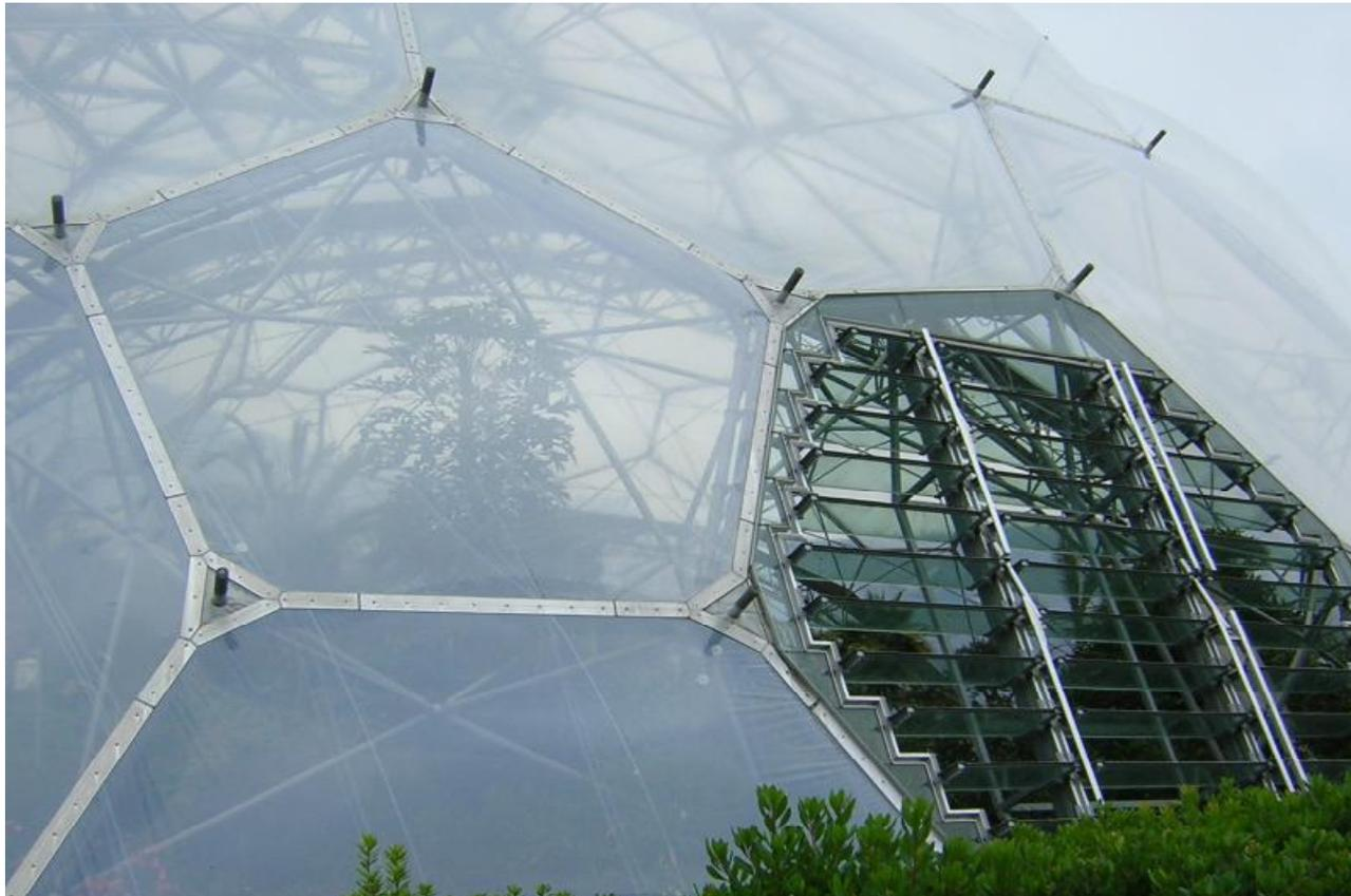
1.11 Up-close look at the transparent glazing of the ETFE pillows and ventilation. Each hexagon (or pentagon) is a slightly different size, allowing the structure to better conform to the site.
